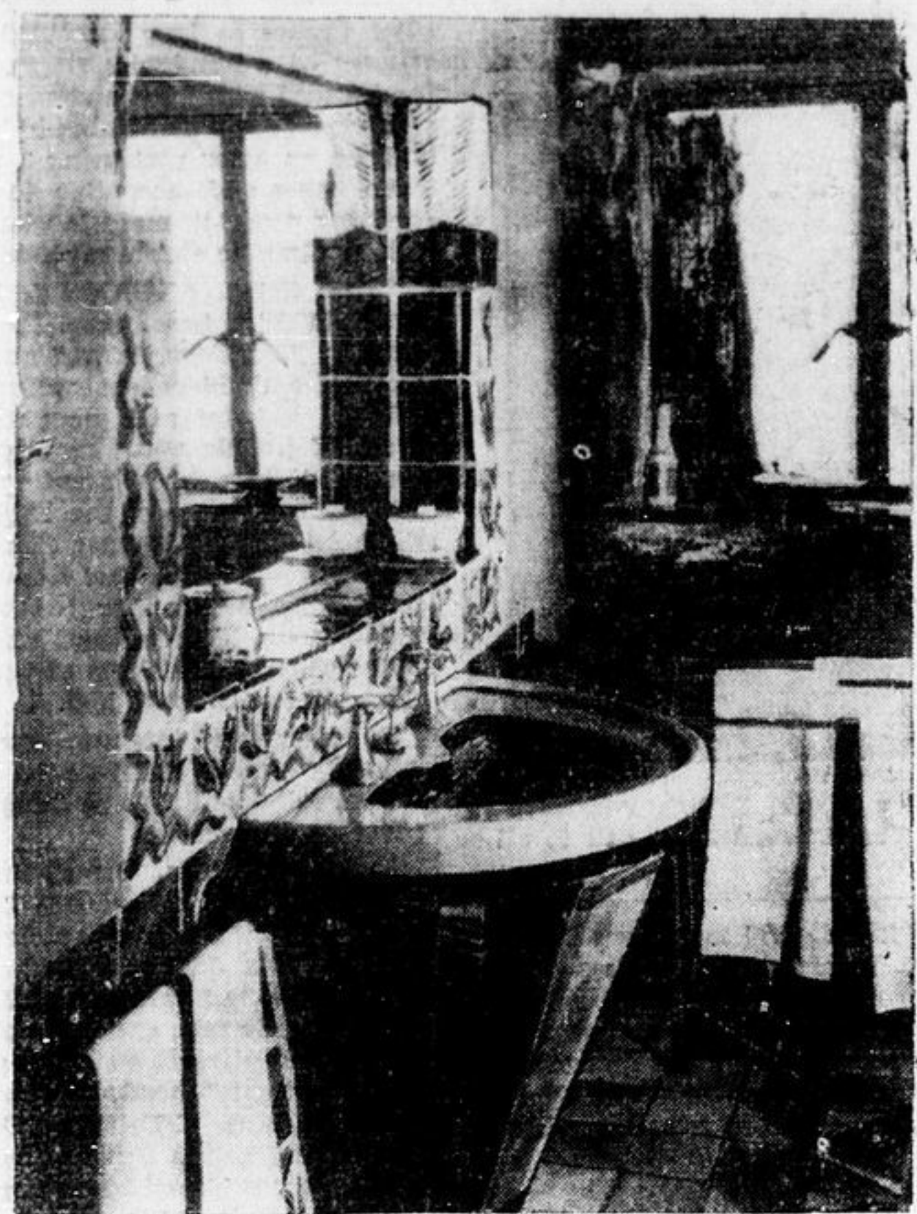
Here is a bathroom with floor, wall tiles and fixtures of tiles hand-made and hand-decorated by Henry Varum Poor, the famous artist, who built his own home on a rocky hillside. This bathroom is in brilliant coppery tones with sepia and black accents.
