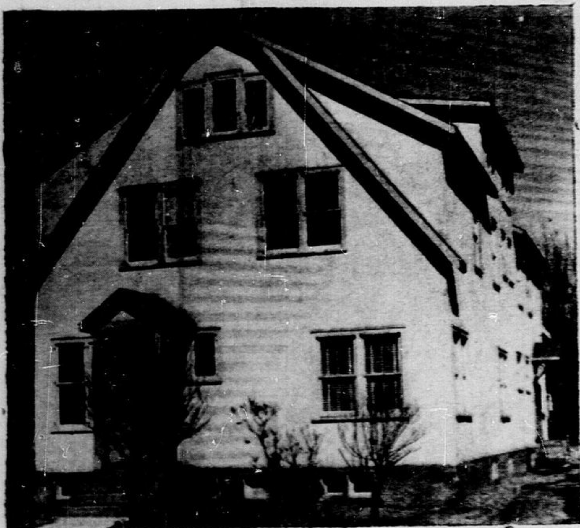
A small house at 108 Spruce Street North, Timmins was converted into this large apartment house by Dave Martin, general contractor. Mrs. P. Richer is the owner.
