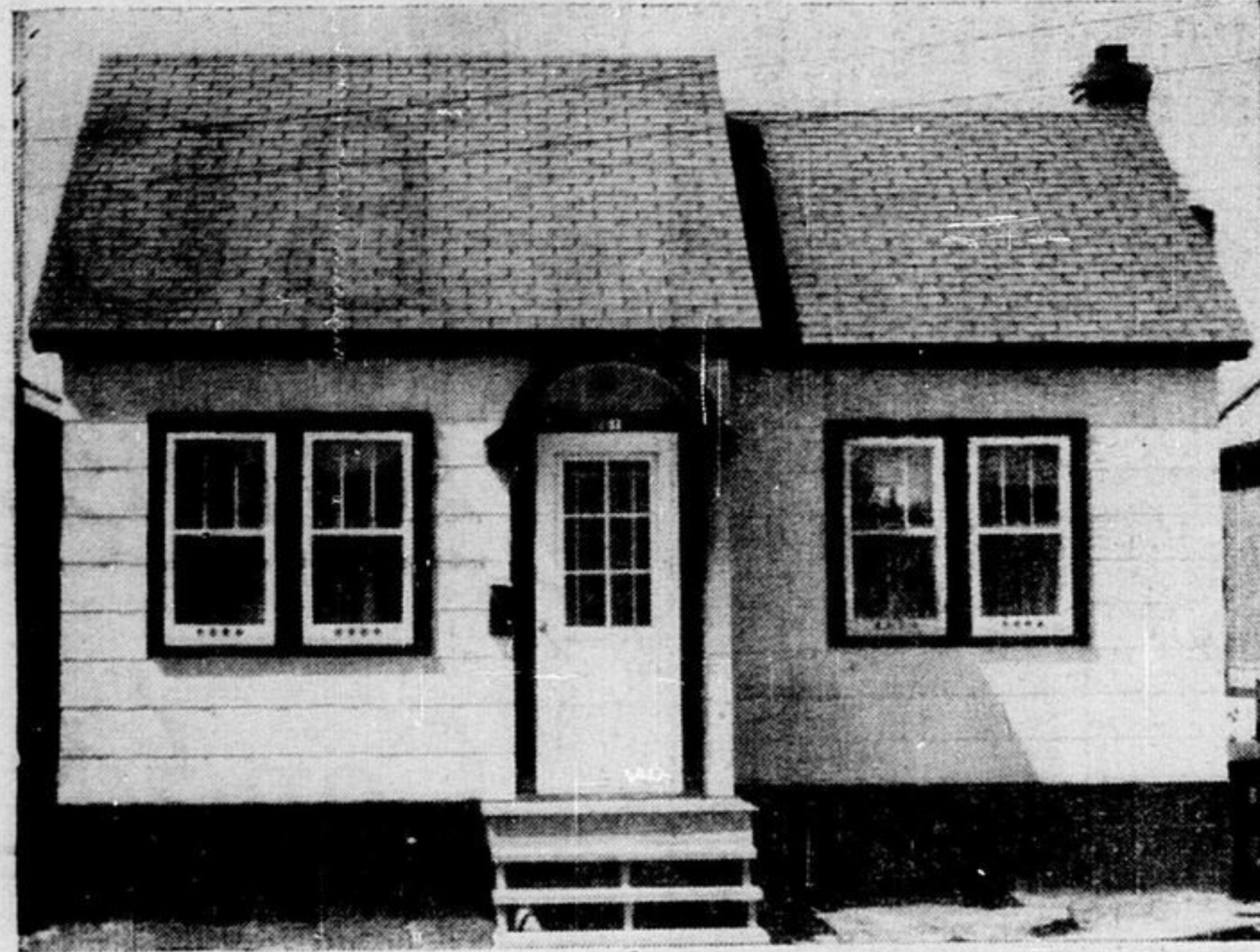
The new home of Mr. and Mrs. John Erickson at 261 Elm Street North, Timmins, shows clearly how pleasing proportions can add beauty to a small dwelling. This building was designed and construction supervised by the George Taylor Hardware. Materials were also supplied by this firm.
