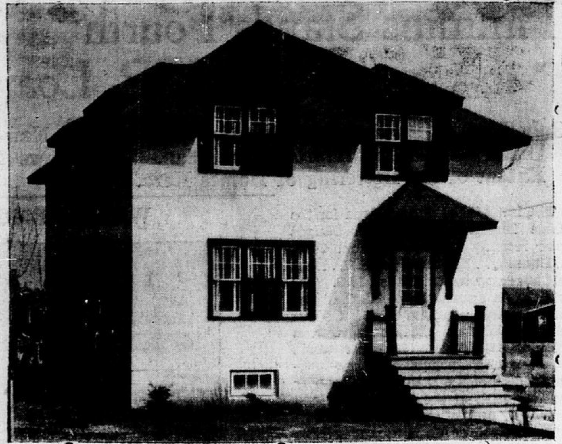
The residence of Mr. and Mrs. T. Rutherford Langdon, corner of Powell avenue and Isabel avenue, South Porcupine was designed by G. D. Hamilton Lumber Company, who also supplied the materials. The broken roof-line is a distinctive feature of the elevation. Advance Photo and Engraving
