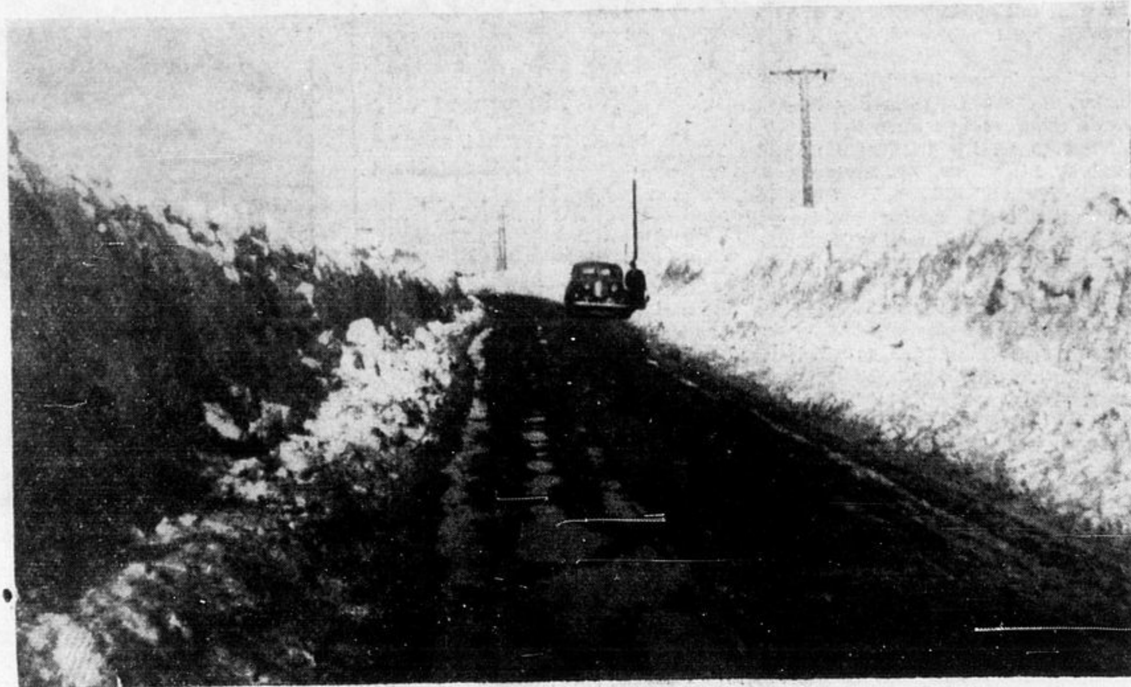
Above is a scene snapped on the highway near Ramore. The snow piled twice the height of the car at the side of the road makes it useless to deny that there was lots of snow in this North this year. It also suggests the credit due to the Dept. of Highways for keeping the highway open all winter, despite the evident difficulty. (Advance Photo and Engraving)
