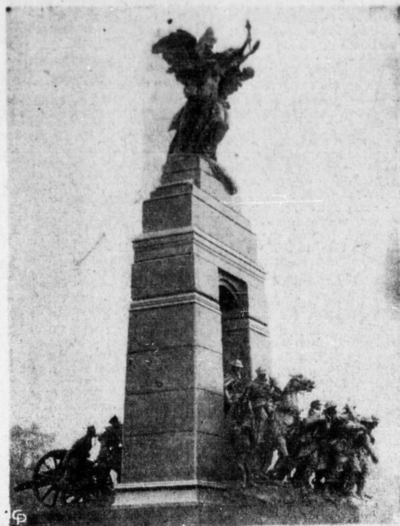
Work on the Canadian War memorial at Ottawa has now been completed. The King will unveil the memorial during his visit to Canada next summer.
