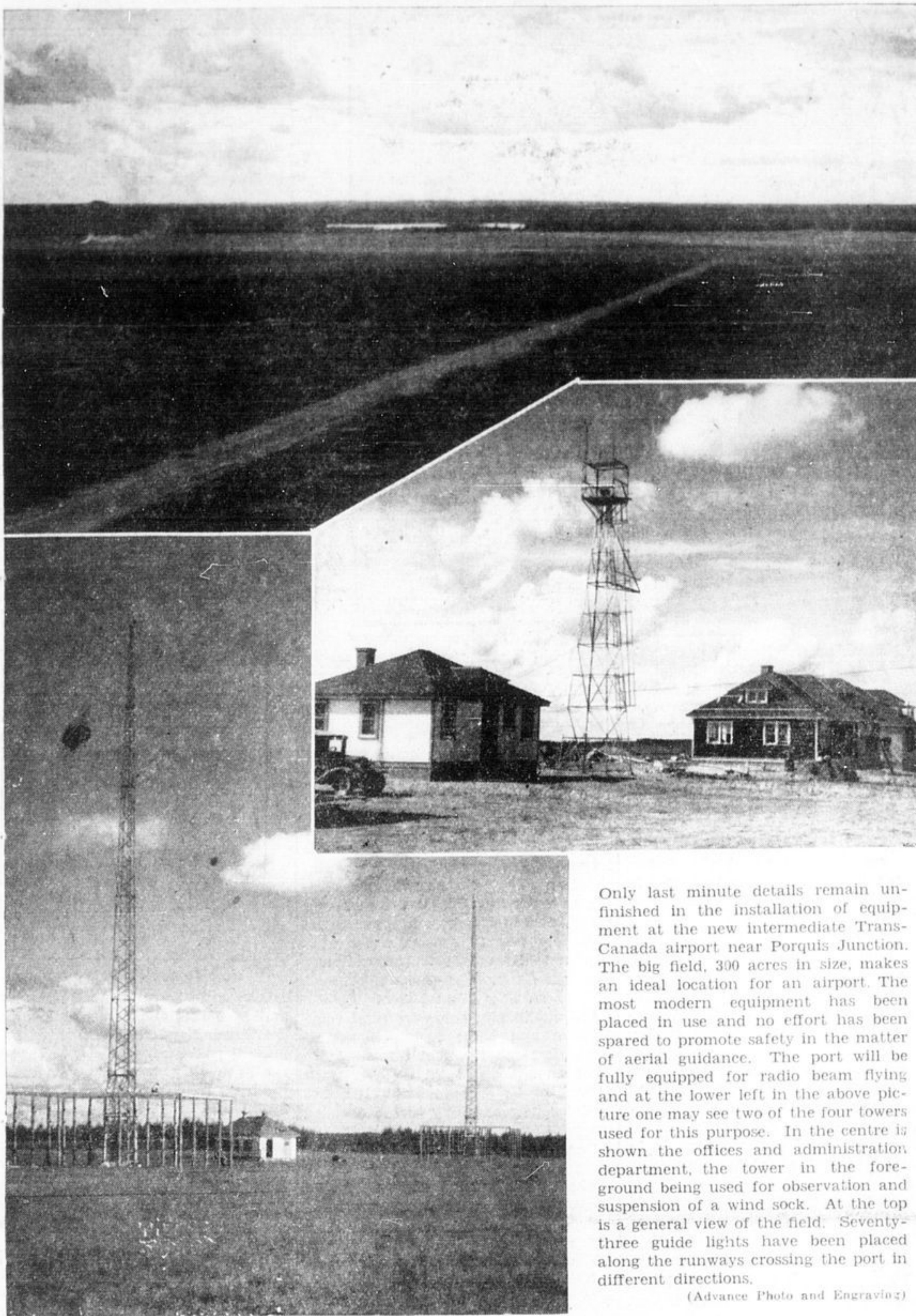
Only last minute details remain unfinished in the installation of equipment at the new intermediate Trans-Canada airport near Porquis Junction. The big field, 300 acres in size, makes an ideal location for an airport. The most modern equipment has been placed in use and no effort has been spared to promote safety in the matter of aerial guidance. The port will be fully equipped for radio beam flying and at the lower left in the above picture one may see two of the four towers used for this purpose. In the centre is shown the offices and administration department, the tower in the foreground being used for observation and suspension of a wind sock. At the top is a general view of the field. Seventy-three guide lights have been placed along the runways crossing the port in different directions.
