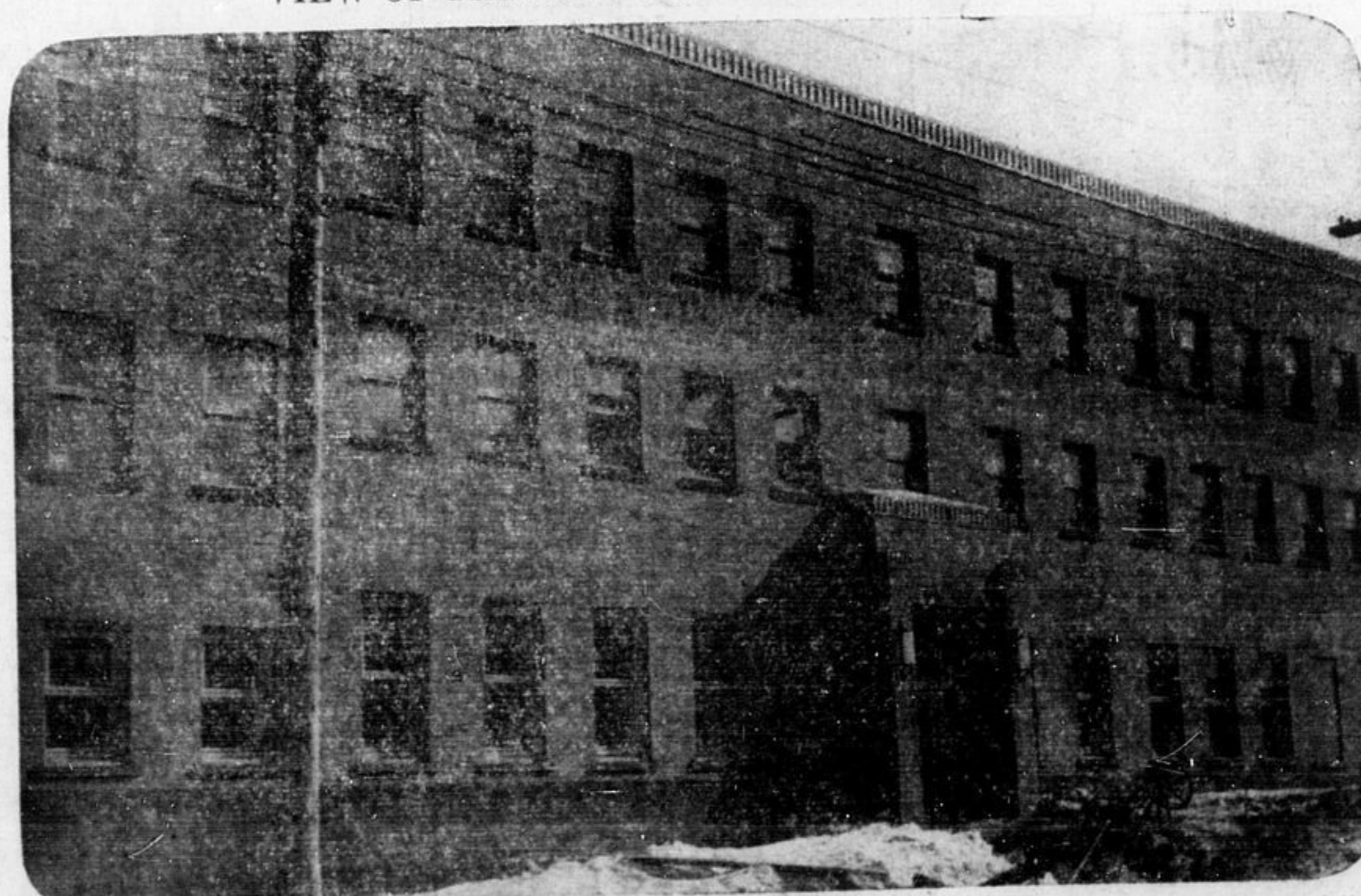
The above photo shows practically all the Cedar Street front of the new addition to St. Mary's hospital. This new wing of the Hospital was formally opened on Saturday, and elsewhere in this issue will be found a full report of the opening ceremonies, as well as a description of the new addition and its various features, together with incidental references to the history of the St. Mary's hospital and its progress.
