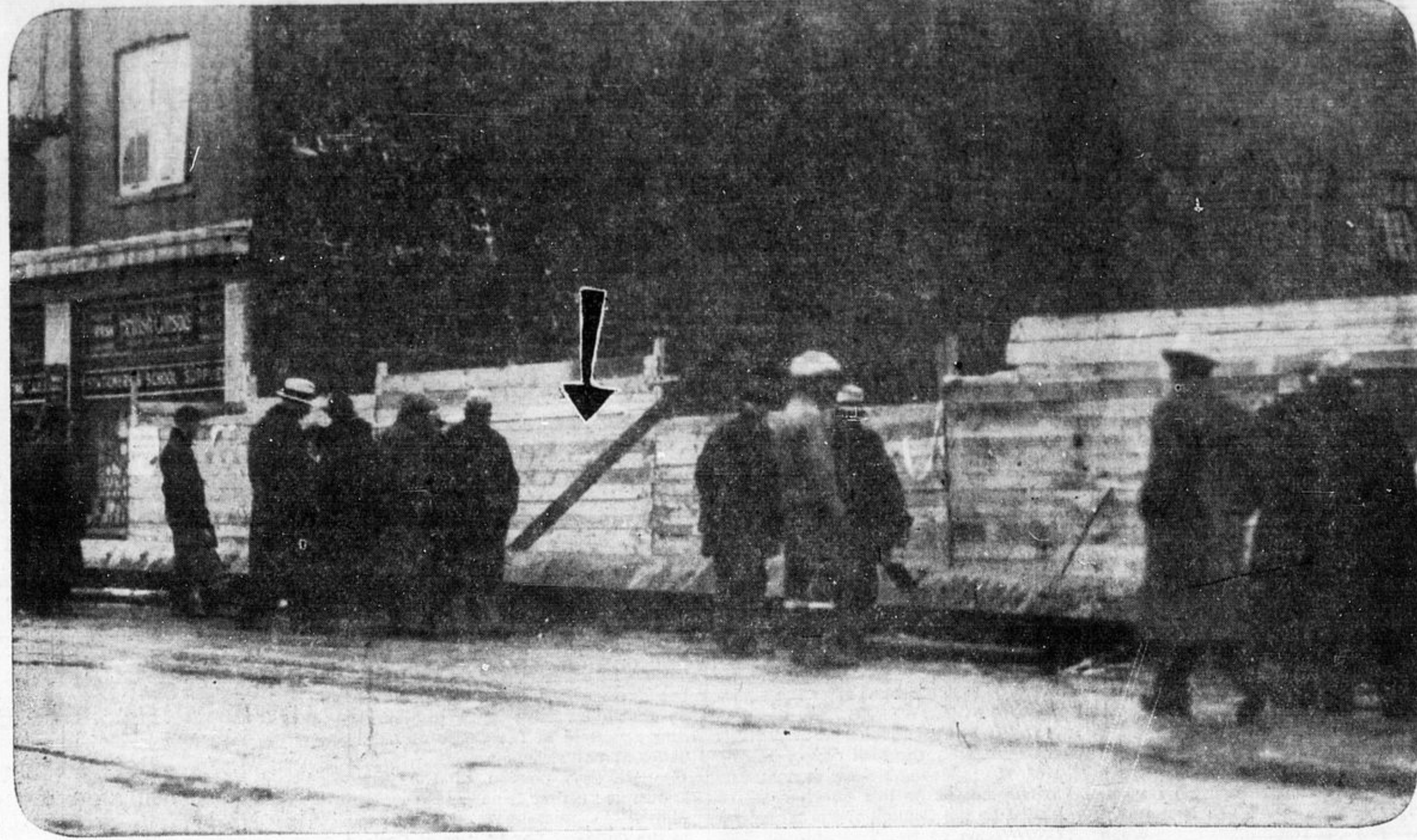
W. R. Randolph, 163 Avenue Road, and George Kepka, 212 Elm Street North, had a miraculous escape from death or serious injury this morning when a steel girder, 50 feet long, crashed into the street from the upper storey of the Bucovetsky building, Third Avenue, which was recently destroyed by fire. Workmen at the time were preparing to take the girder down, which was the last piece of the superstructure remaining in position. The two men who were standing chatting at the time jumped clear but not before both were grazed slightly. The picture above shows the heavy beam after falling in the street, demolishing a wooden barricade and two electric light standards in its path. One of the men was still crouched under the leaning barricade when workmen rushed to the scene and assisted him to safety. The arrow points to the position where the two men were standing.
