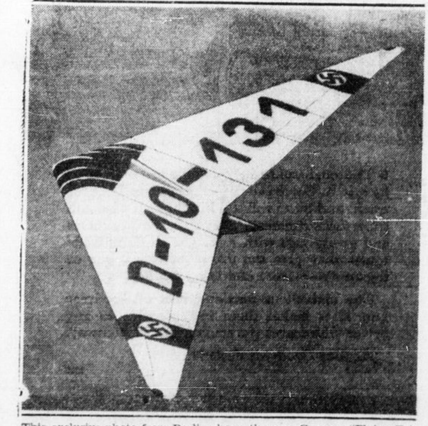
This exclusive photo from Berlin shows the new German "Flying Triangle" in its best flight on August 30. The tail-less plane, which developed a speed of 145 miles per hour with a midge motor of 80 horsepower, can also be used as a glider. It was constructed by a German Air Force Lieutenant.
