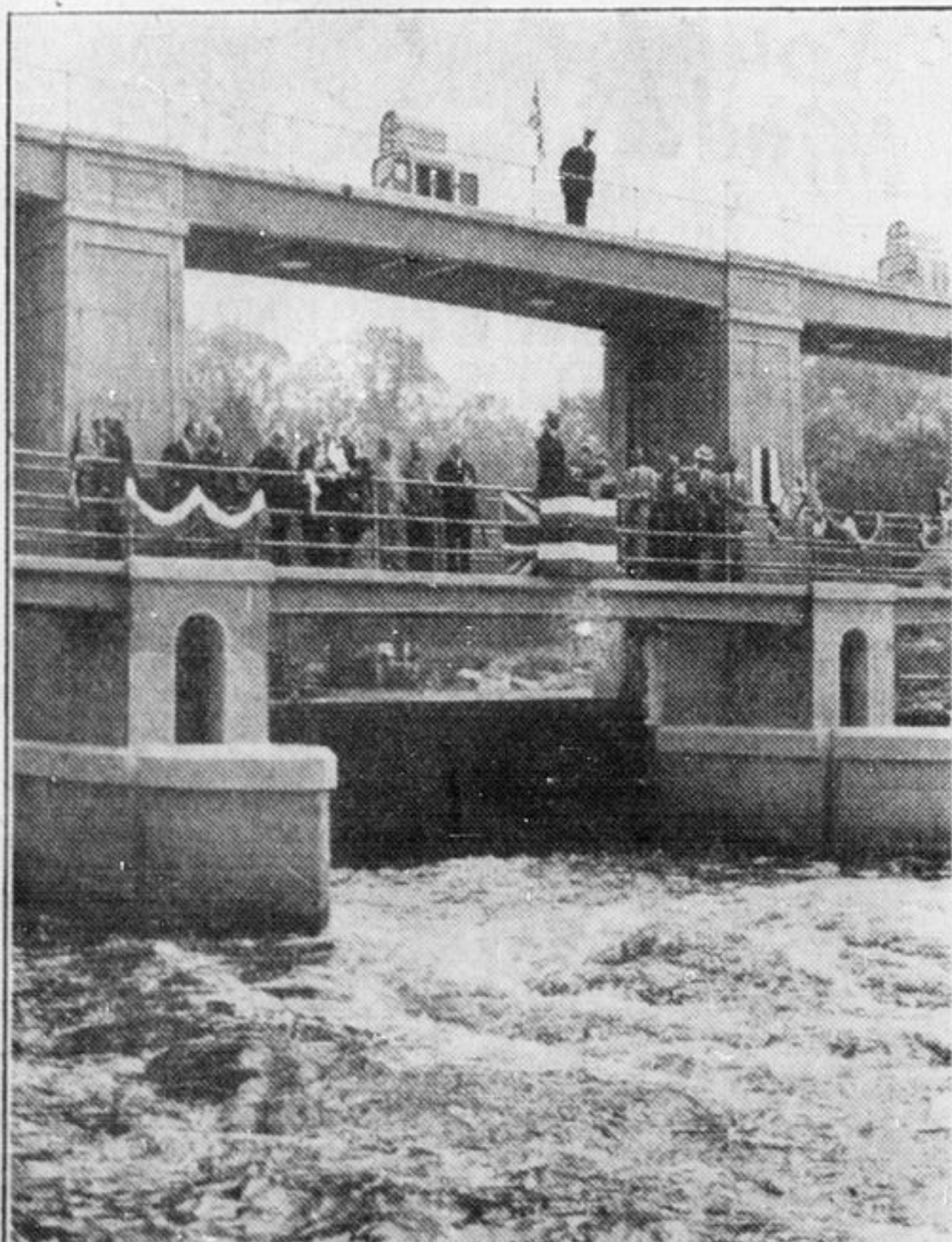
A general view of the opening of the tidal sluices at Allington Locks, Maidstone, Kent, by the Right Hon. W. S. Morrison, British Minister of Agriculture. The sluices have been constructed as part of a comprehensive scheme for flood alleviation in the Medway Valley.
