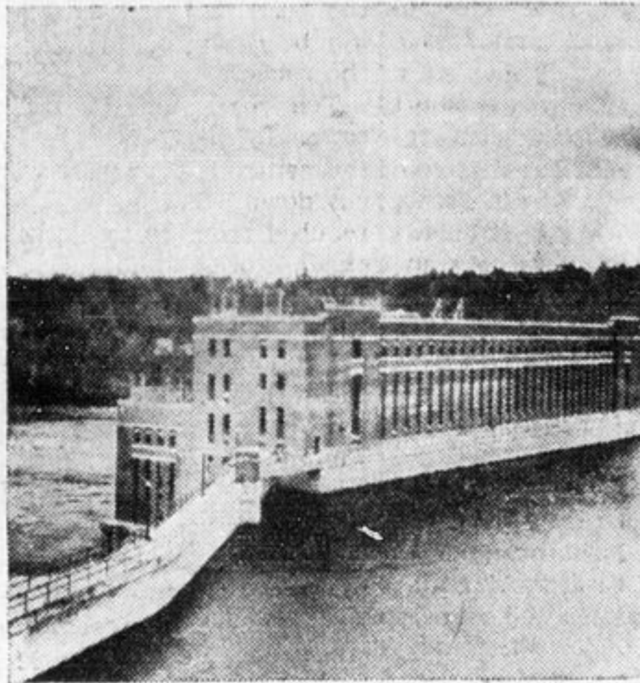
LaGabelle Power Plant of Shawinigan Water & Power. Gongs were fed by "Canada's Biggest Cook."
