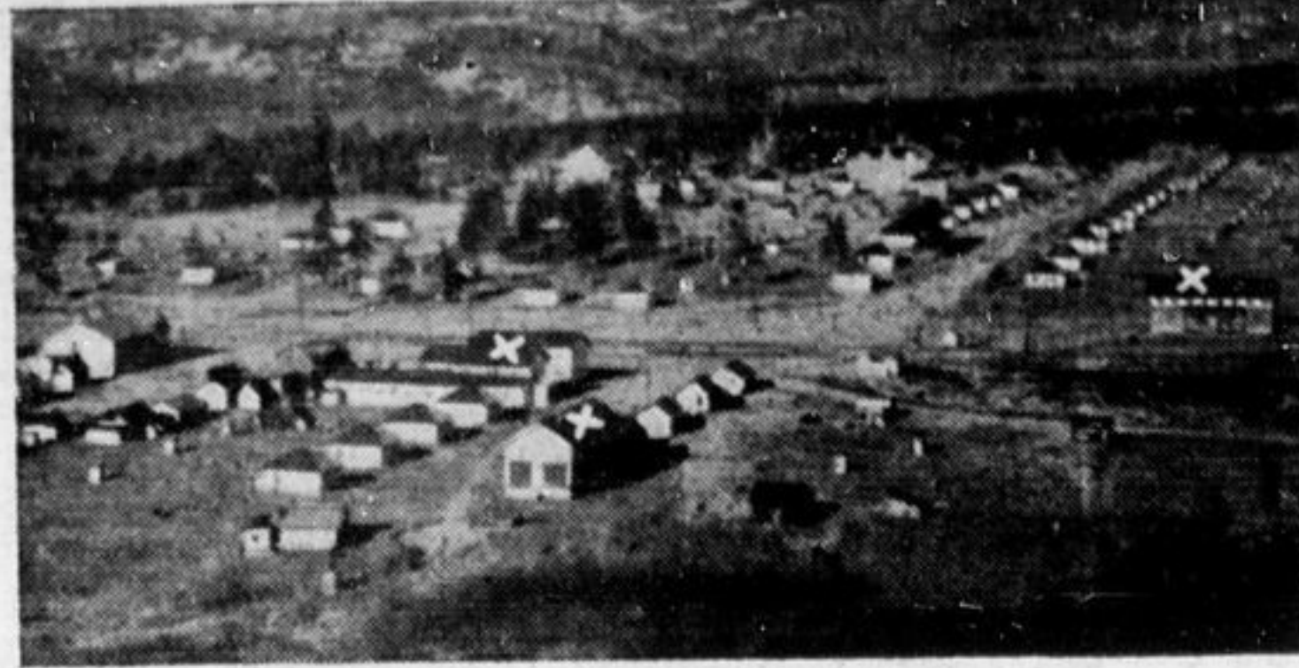
An International Nickel Co. town—Levack, Ont. Boarding houses we operate for the Company are marked "X."
