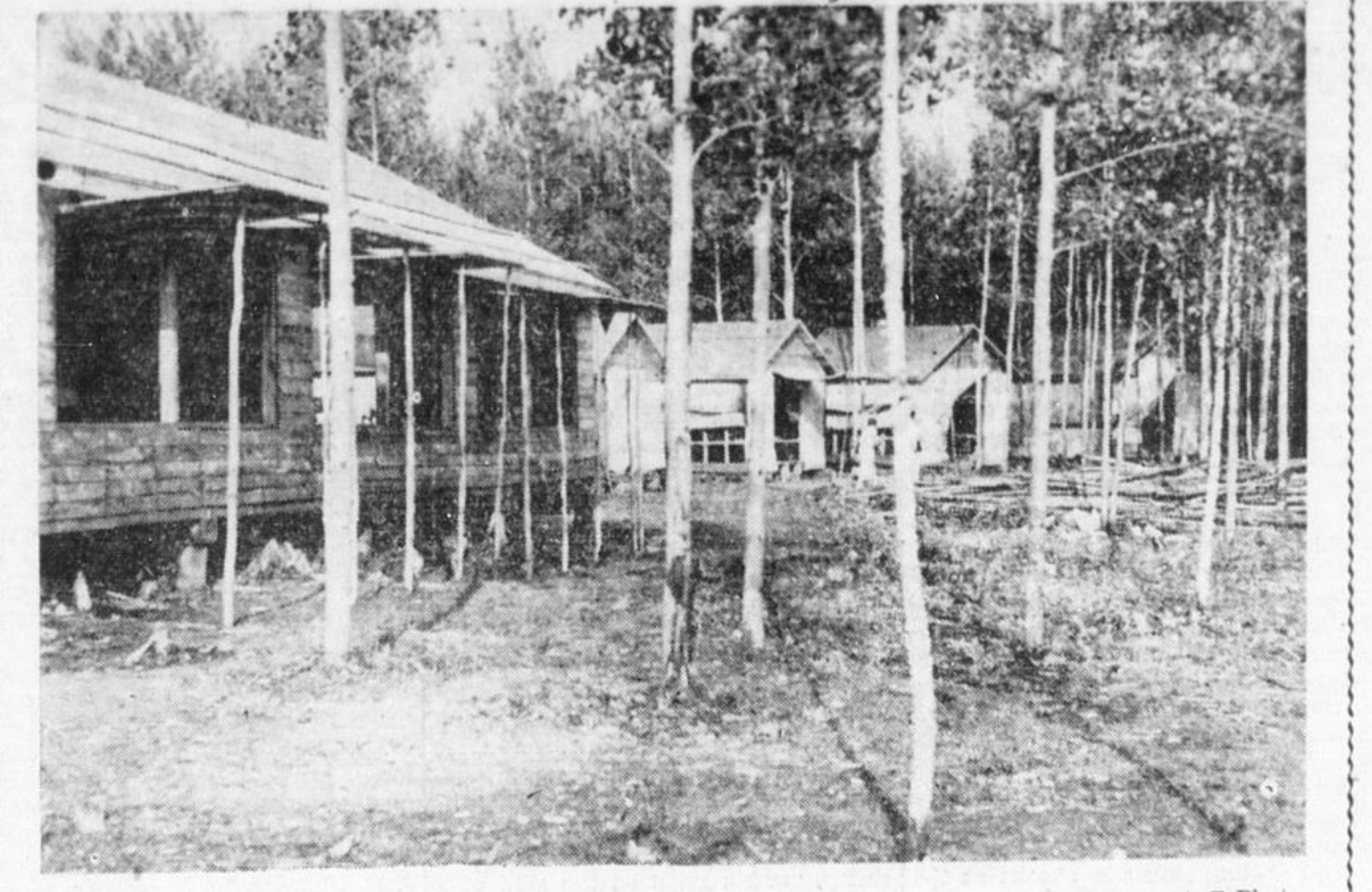
—Advance Staff Photo The buildings at Camp Waskesu on beautiful Nighthawk lake are shown in the above photograph. At the left is the cookhouse and dining pavilion and to the right may be seen four of the five sleeping huts that face the lake. Though the dining hall is partially screened, the huts are not, for mosquitoes and flies are kept far inland by the steady breeze from the lake. P. T. Moisey, of Timmins as camp leader, supervised the activities of forty Cochrane district Tuxis boys and Trail Rangers here a short time ago, and has been the leader in the movement to build up the camp from nothing with the help of the boys of Excelsior Tuxis Square of the Timmins United Church.
