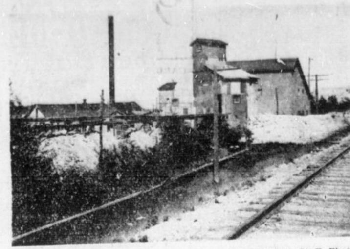
Advance Staff Photo Here are the buildings of the Gillies Lake-Porcupine mine (formerly the ment for milling 60 tons of ore daily. New Denver flotation cells, installed in the mill building shown at the right, will put the mine on a paying basis it is expected. A four-foot vein of high-grade, found in sinking a winze from the 500-foot level, is producing a considerable amount of the mine's pay ore now.
