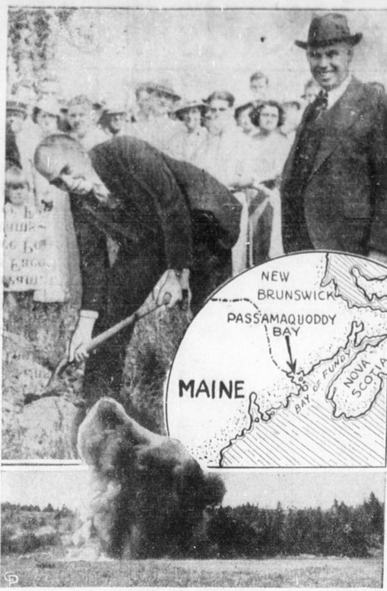
Work starts on the U.S. Government's $30,000,000 Passamaquoddy tidal power project as Major Philip E. Fleming, army engineer in charge, breaks ground at Eastport, Me., while Rep. Ralph Brewster and crowd looks on. Project will harness famous tides of Bay of Fundy for electric power. Lower is first blast set off by telegraph from Washington. Map shows location of project that will employ thousands for several years.
