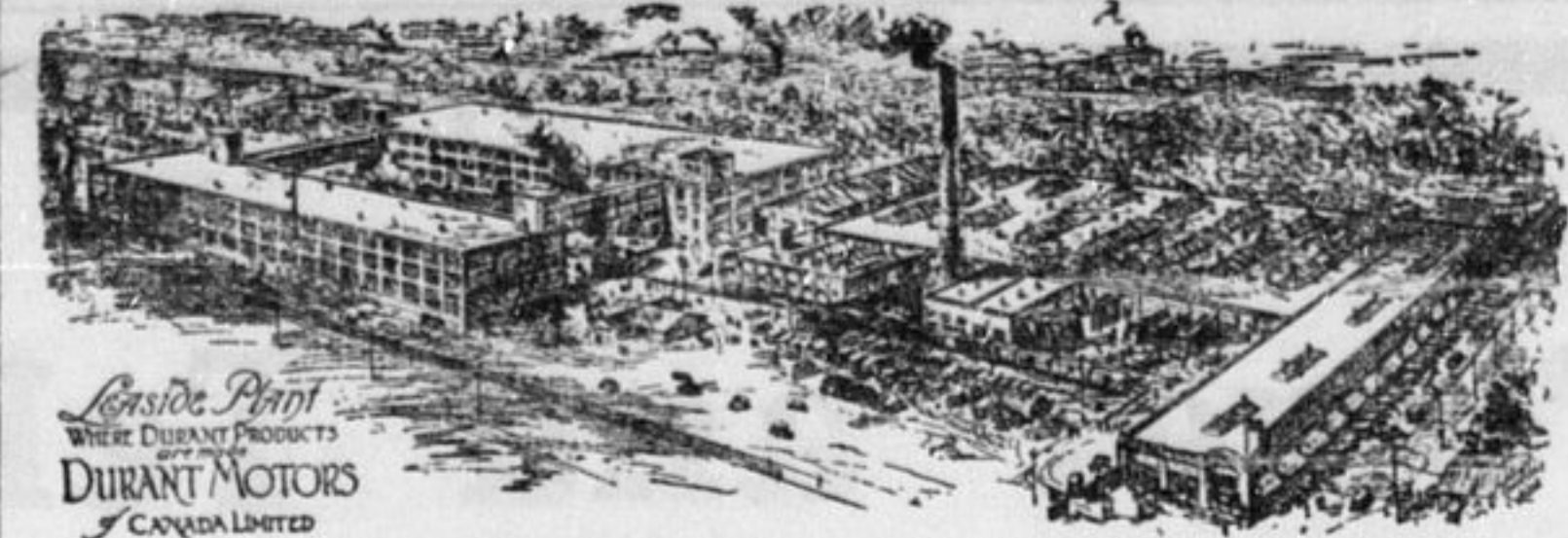
An airplane view of the plant of Durant Motors of Canada, Limited at Leaside, on the outskirts of Toronto. The plant covers nearly 15 acres and has approximately half a million square feet of oor space. It is modern in every respect and has a capacity of upwards of 175 cars a day.
