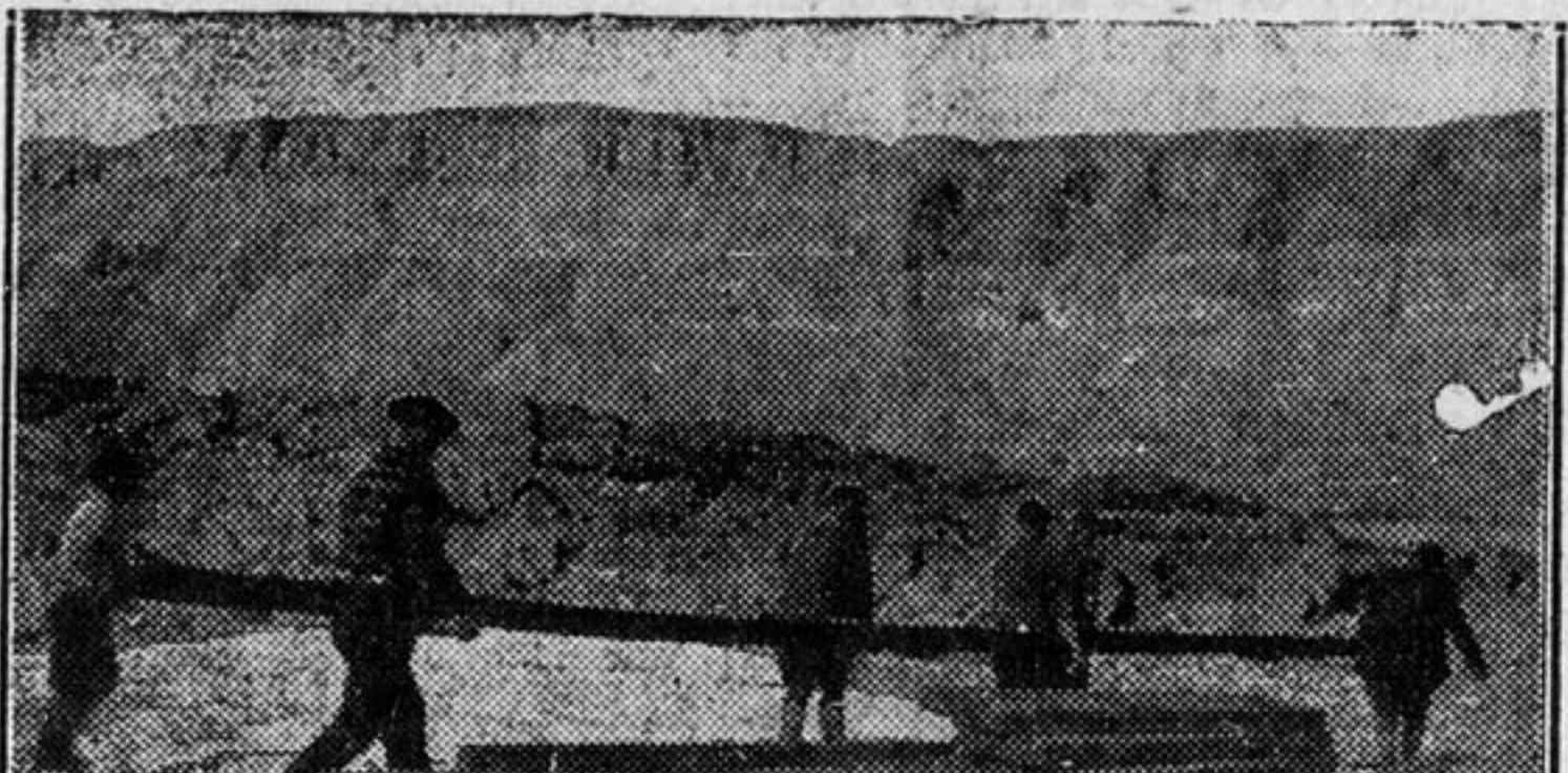
Mr. George P. MacKenzie, three members of the R.C.M.P. and a native carrying timber for the foundation of the new government building.
