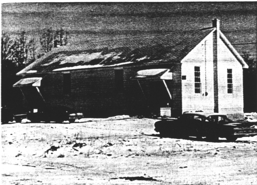
The New Coldspring Longhouse near Steamburg, 1968.
