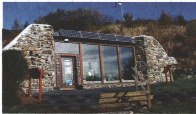
A sample Earthship similar to what Fran's will look like with south facing wall of windows to allow for food growth inside
