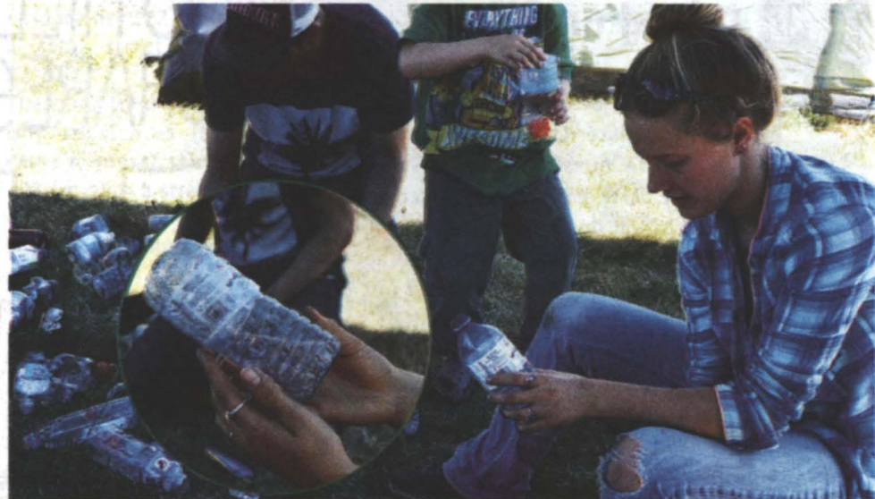
Plastic bottles are being recycled, cut and put back together to form bottle bricks to go in between concrete bringing light into the house.
