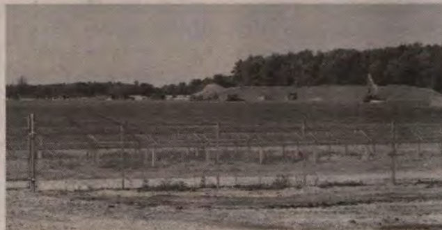
First Solar already has frames in place. (Photo by Chase Jarrett)
