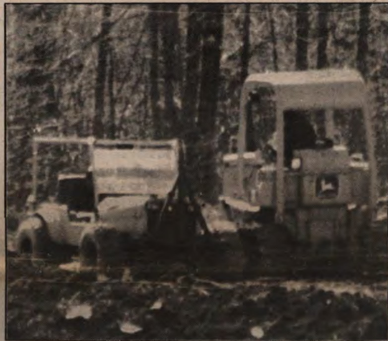
Workers at proposed tire recycling plant before HED protest halted construction.
