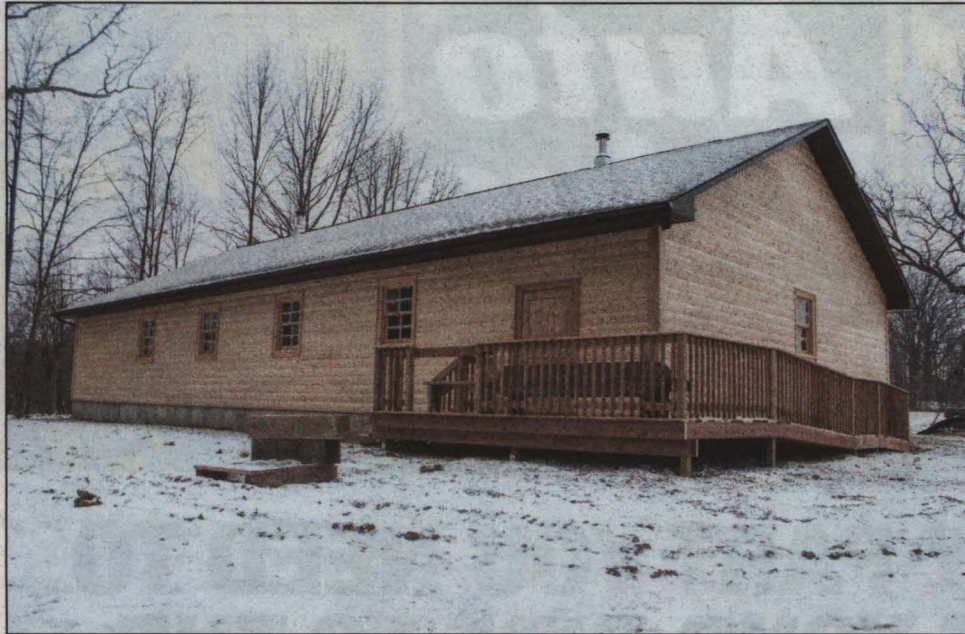
A view of the new longhouse from the mens door - even this far away from the building, the scent of pine and new home lingers in the air. PHOTO BY CHEZNEY MARTIN
