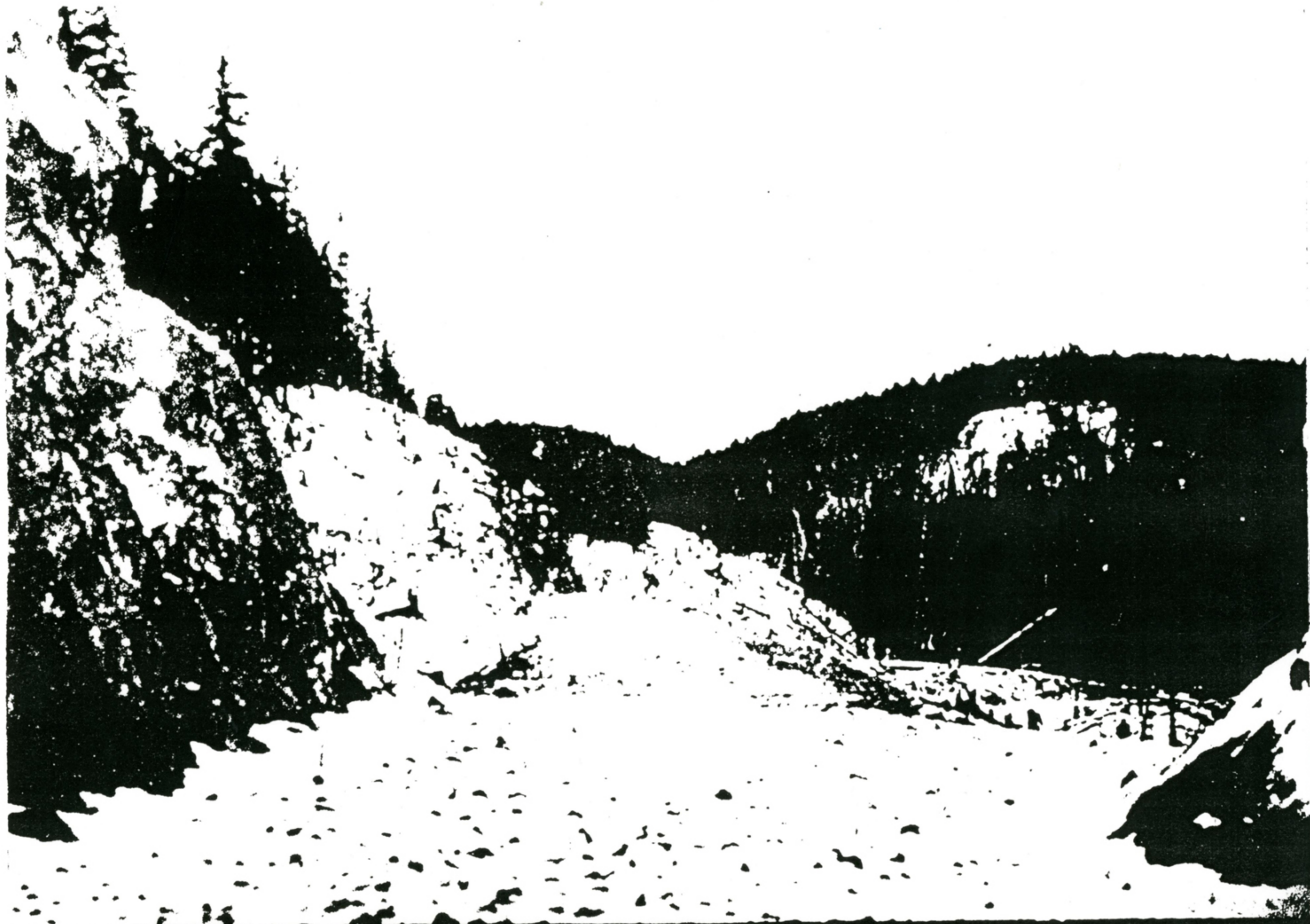
ROCK WORK ON J. ISBISTER'S C. P. R. CONTRACT
