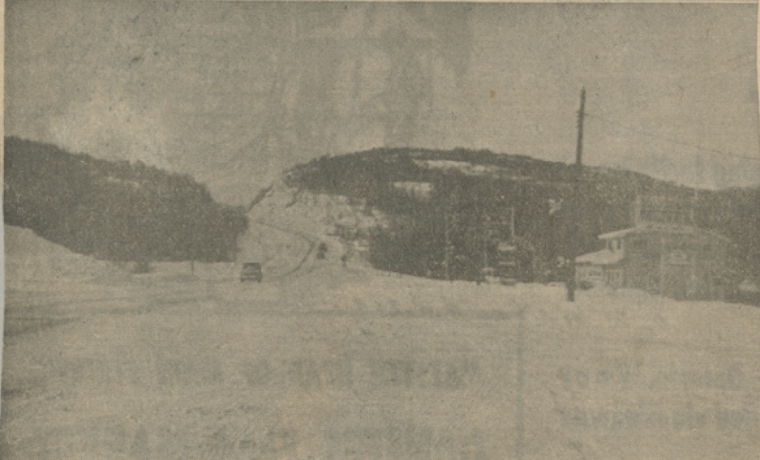
ROADS IMPROVING —Roads remained curving and steep along the north shore of Lake Superior while much of the work had to be done by hand as seen in the TOP PHOTO. Conditions today (BOTTOM PHOTO) are different as both the hills and curves are much more gradual. —Photos from Inez McCuaig
