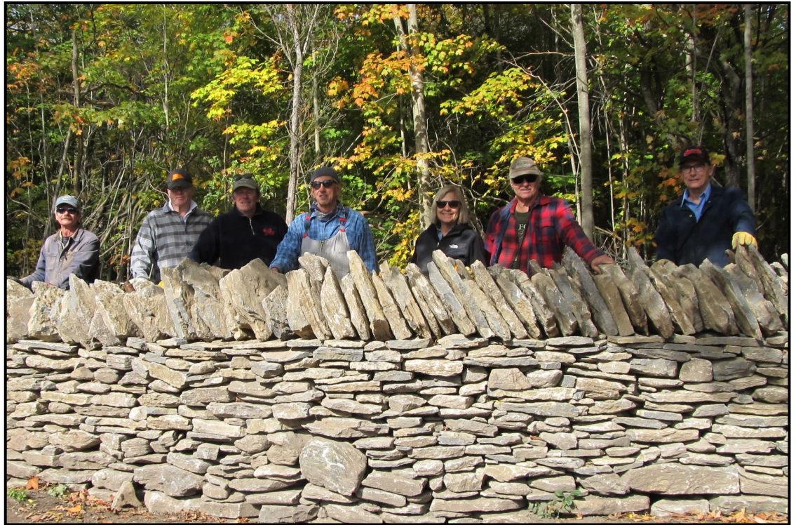
Each rock in building a dry stone wall is lifted on average four times. Many weigh 50 lbs (110 kgs) or greater, but others used as “hearting” rocks are smaller, so building a wall is a testament to many hands making light work. From the left: Greg Forbes, Tom Foulds, Howard Whittaker, Brian O’Donnell, Anne Dumbrille, Les Stanfield and Joe Keogh.— Mirror Photo
