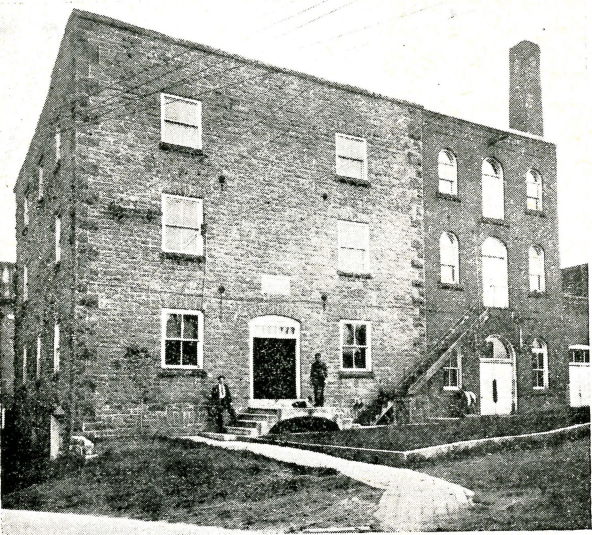
Exterior View of Waterworks Power House
