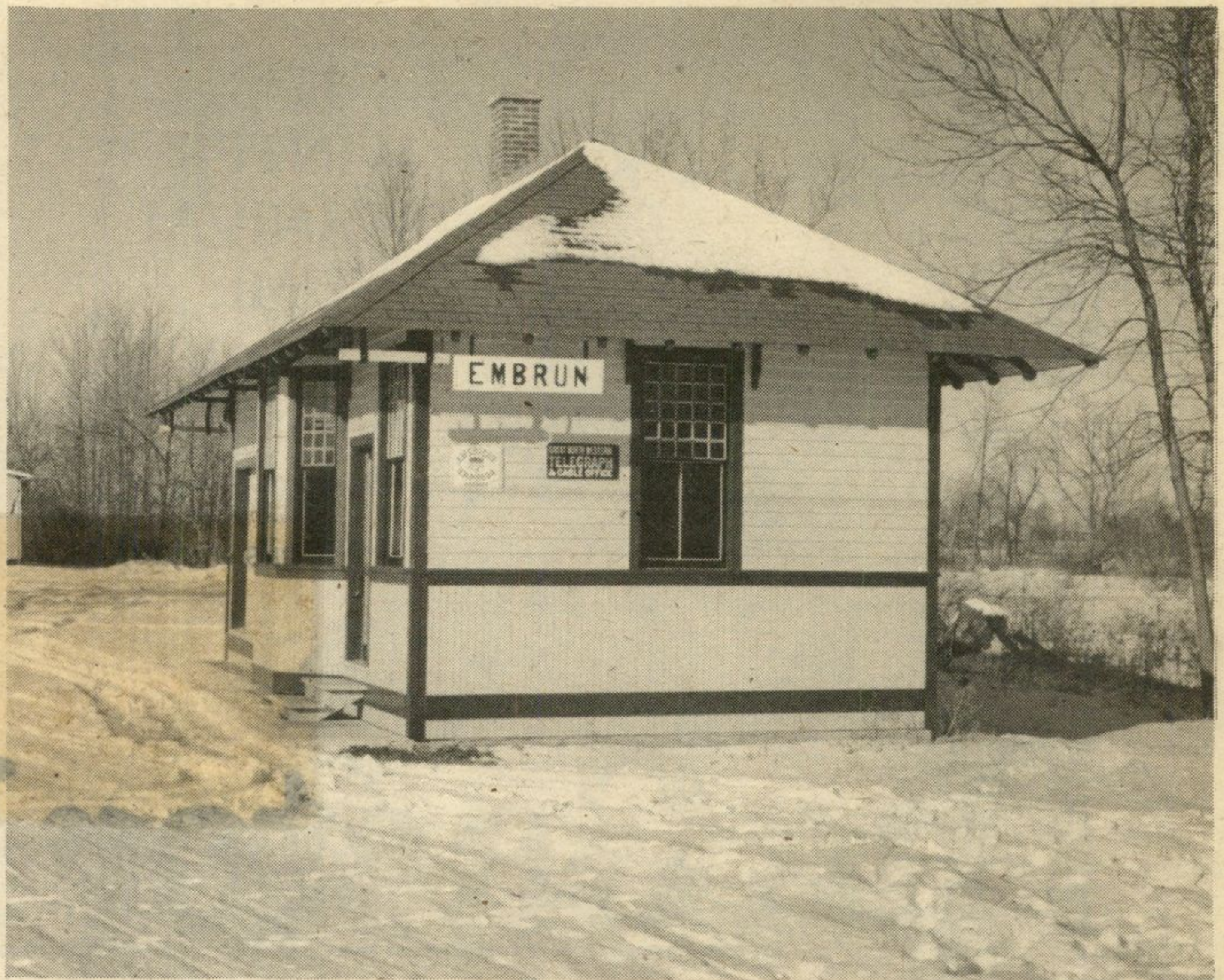
The Berwick Station, pictured above, is one of the projects adding to Russell Township's financial difficulties. Estimates for completing the renovation of the Station are running about $6,000 over-budget. (See story this page).
