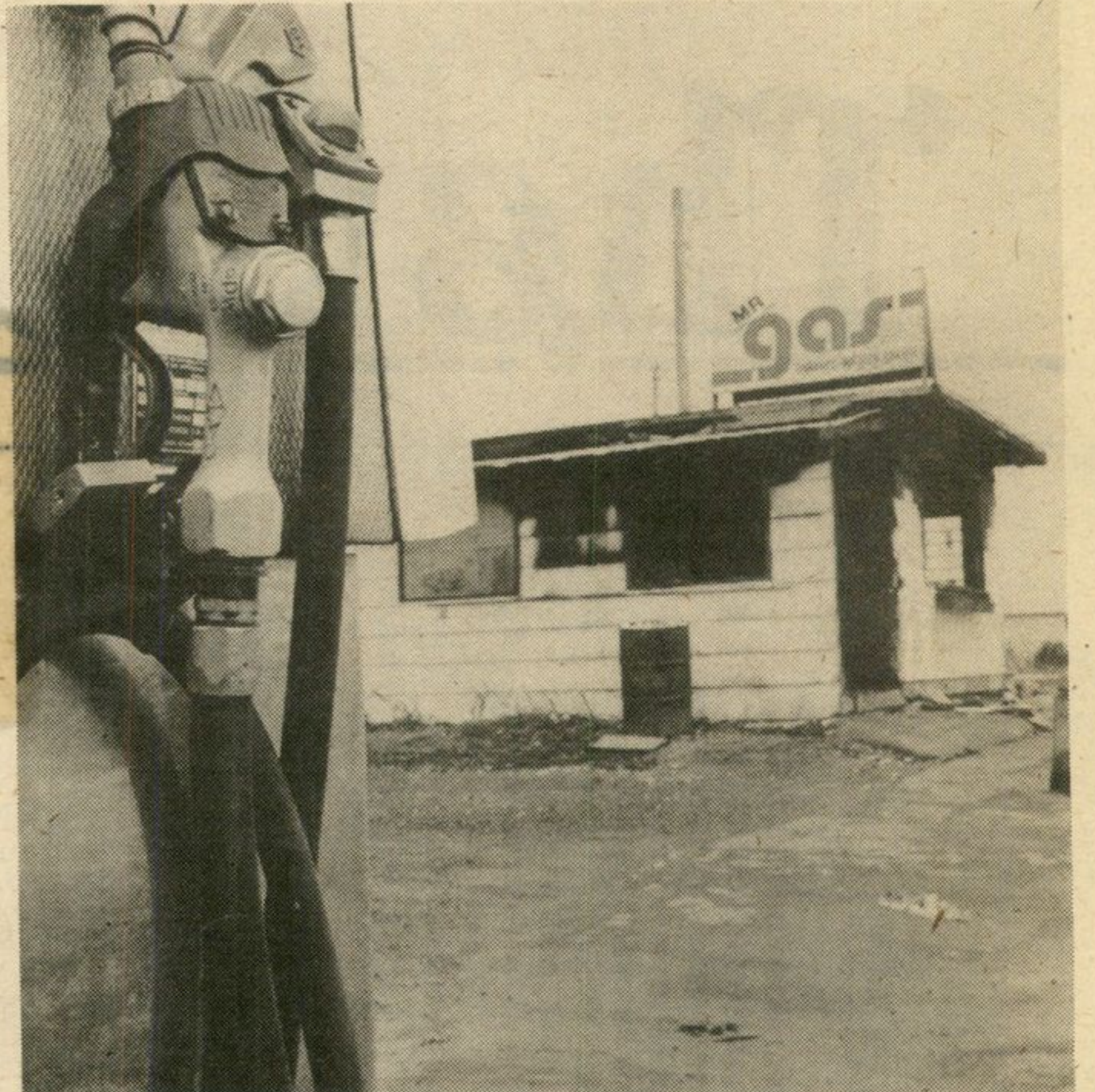
All that's left of the Mr. Gas filling station at the Corner of the Regional Road through Metcalfe and Highway 31 is a burnt out building and locked gas pumps. But it'll be back in operation soon. The Township of Osgoode Council decided to let the company use a trailer on the site. Mr. Gas has promised to submit plans for a new building within six months.
