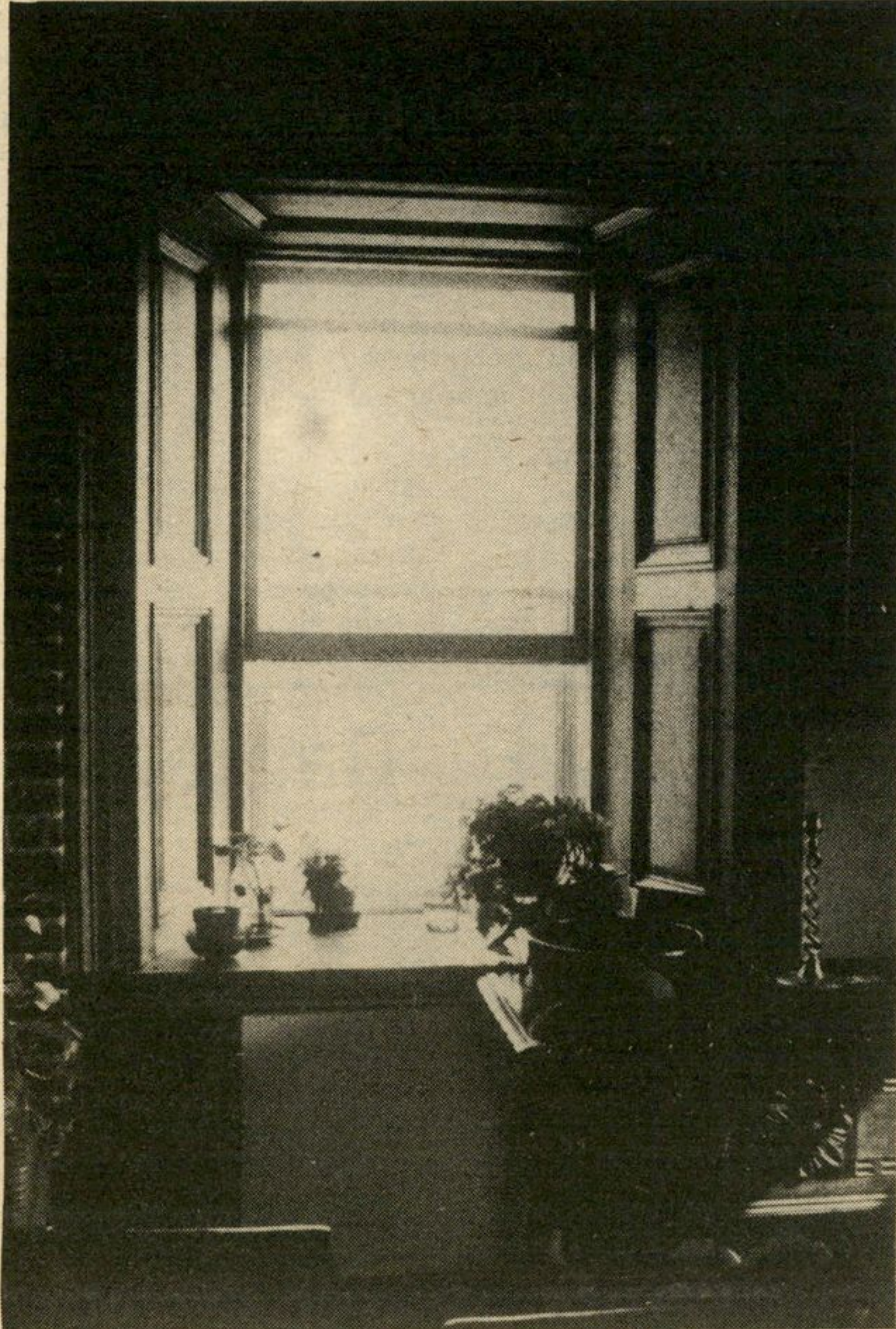
Restored, recessed window. Pine sill is 30 inches deep. (Paul Rodier photo)
