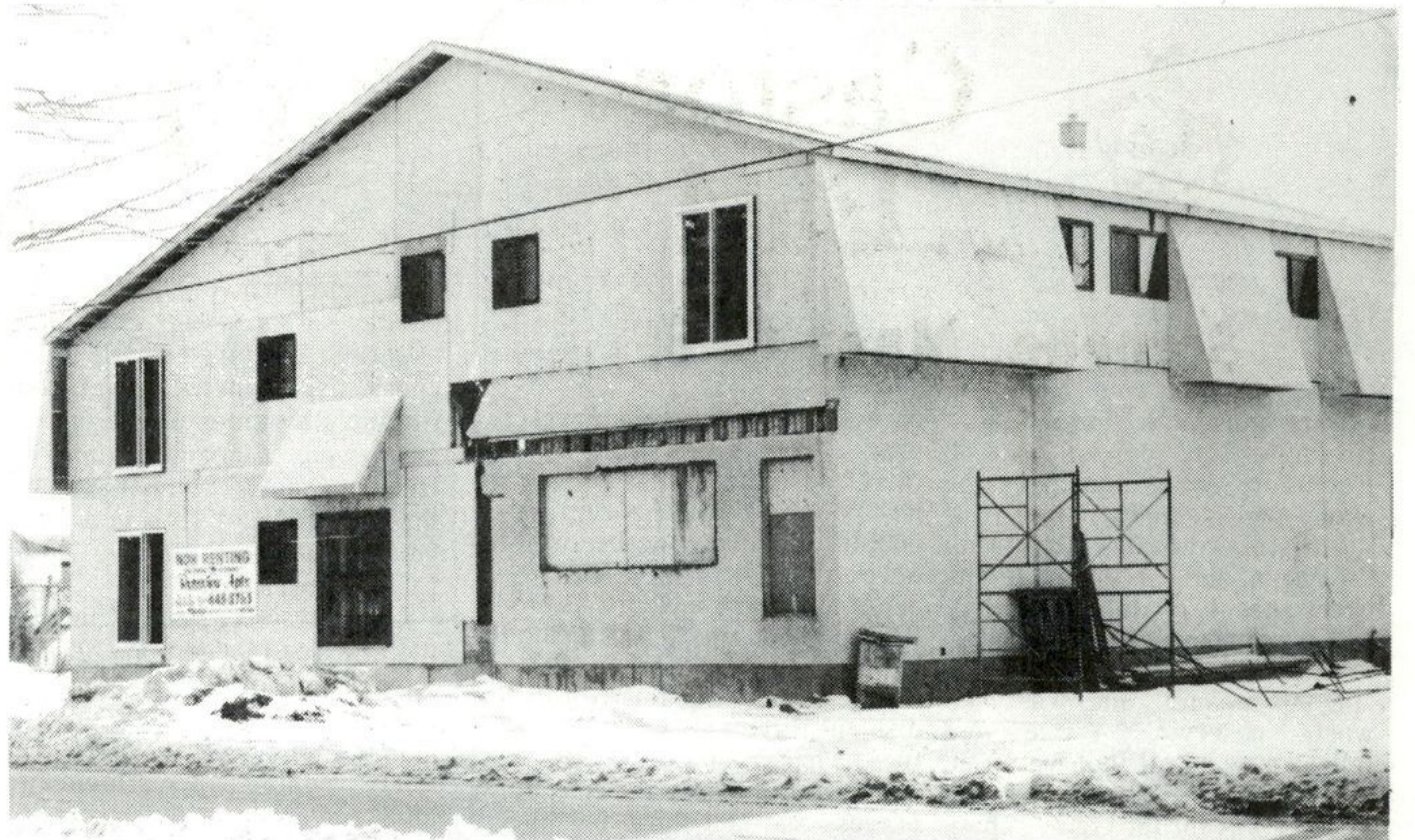
NEW RUSSELL APARTMENT BUILDING
