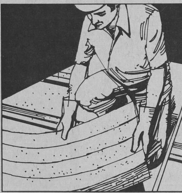
C.M.H.C. no. 6281 FIBERGLASS INSULATION Friction Fit Batts
