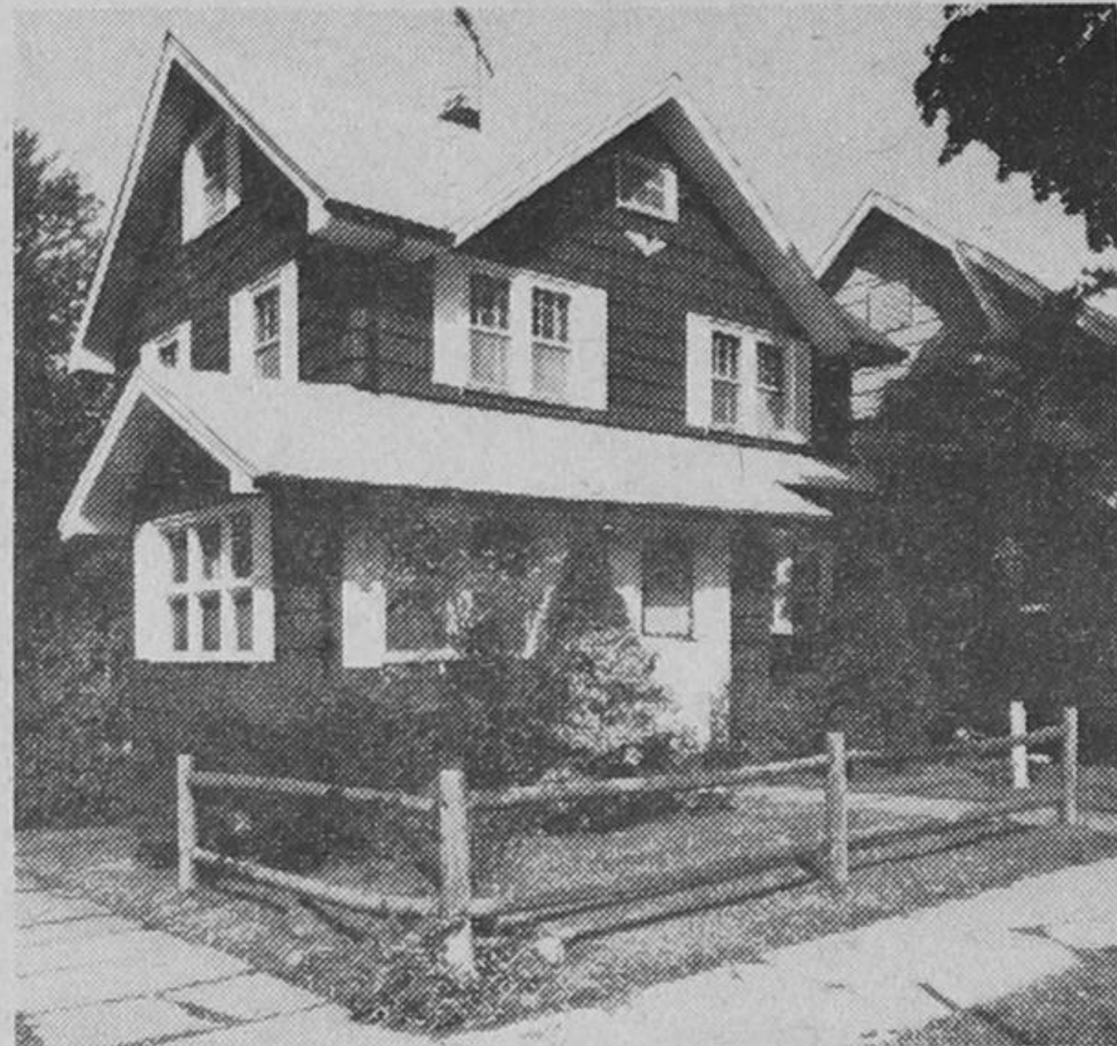
REDDISH ALUMINUM SIDING with an embossed cedar shake finish rejuvenated this older house and eliminated the need for periodic repainting. Contrasting pre-finished white aluminum trim and accessories (storm windows and doors, shutters, soffit, fascia, gutters and downspouts) define lines of the house and add character. New colors and textures baked into the aluminum panels remain attractive up to 40 years and more.
