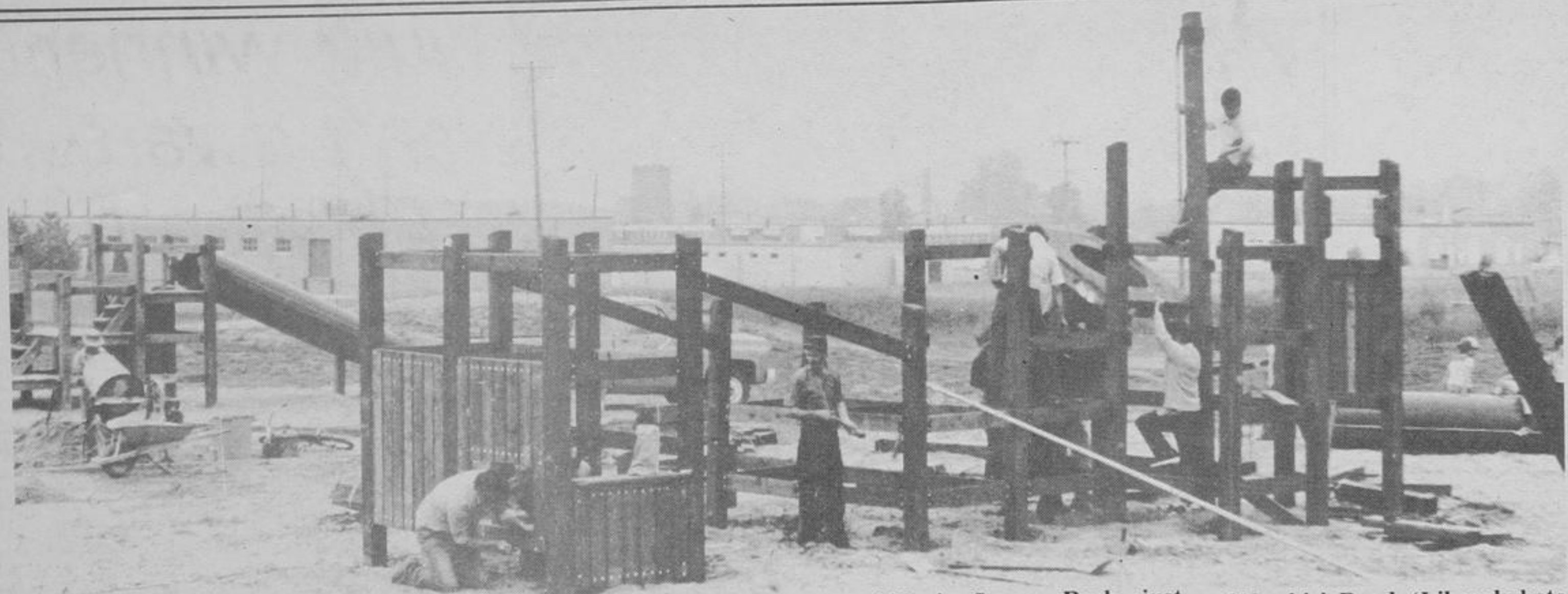
Residents, staff and elected representatives were all out working Saturday morning to construct a creative play area for kids in Sussex Park, just north of Centre Street and east of Newkirk Road. (Liberal photo by Shaaron Hay).
