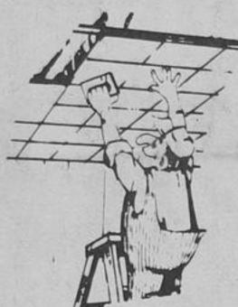
These strong ceiling tiles are ideal for use in any rec room, bedroom or attic. The 12" x 12" x 1/2" tiles have tongue and groove joints which makes application easy and conceals nails or staples. C.M.H.C. approved. 64 tiles per carton.
