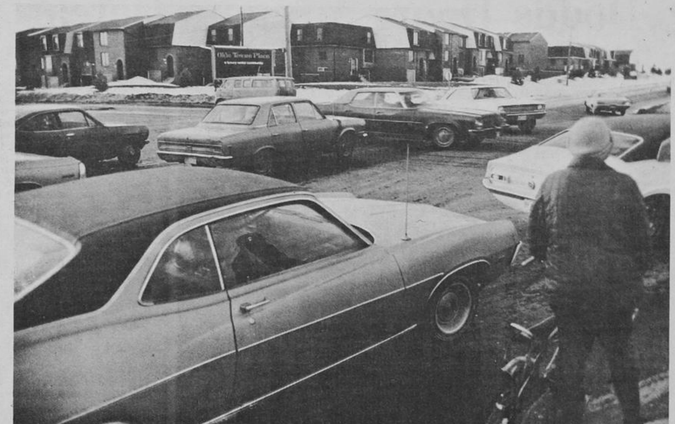
Described as too dangerous at rush hours for a single traffic control officer is this new Thornhill intersection at Steeles Avenue and New Leslie Street. In the foreground several lanes of cars are shown leaving Metro's newly opened extension of Don Mills Road while a bewildered cyclist wonders what to do next. Large numbers of new residents are moving into the new Thornhill development area shown across Steeles Avenue. There have been many complaints of snarled traffic and accidents. (Photo by Susan Samila)
