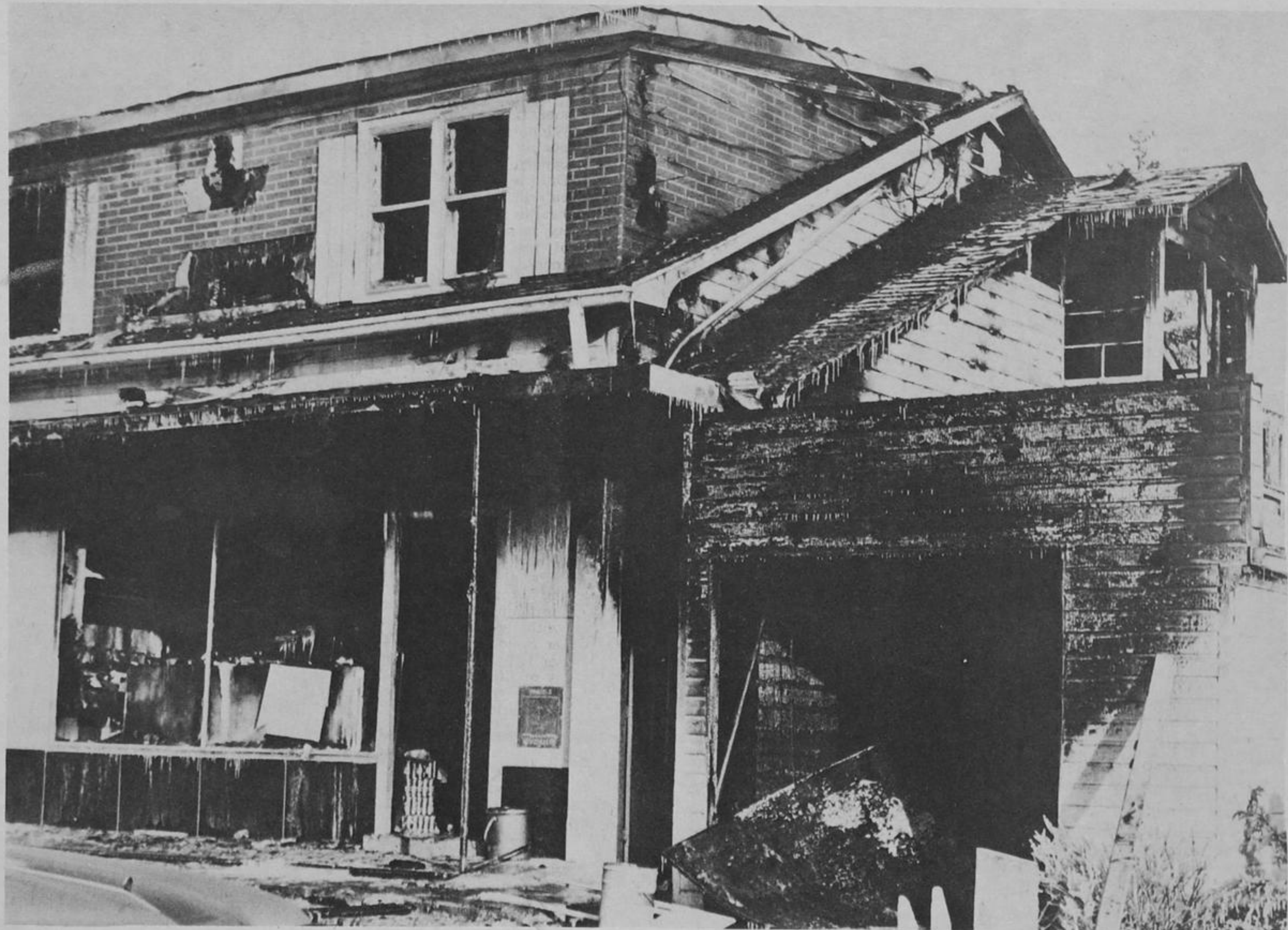
Fire of unknown origin swept through the Pine Grove Market, Campbell Avenue in the Pine Grove area of Vaughan last week, causing more than $4,000 damage.
