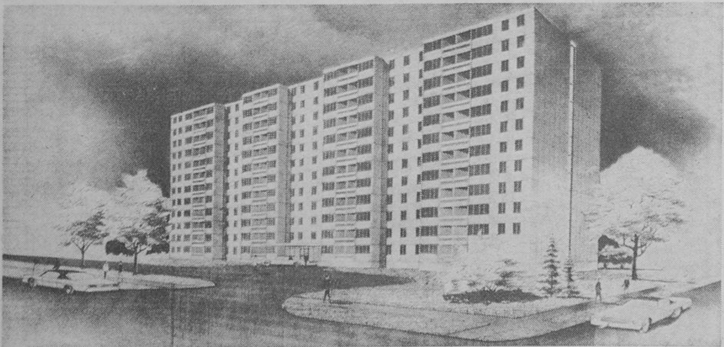
Depicted in this architect's drawing is what may be Canada's first multi-storied structure using a fully integrated, industrialized modular concrete building system. The 12-storey, 184-suite apartment building is to be constructed in Scarborough by Jespersen-Kay Systems Limited after its new plant located in Whitchurch Township goes into production. Construction of the new plant is proceeding on schedule and it is expected to go into production in December.
