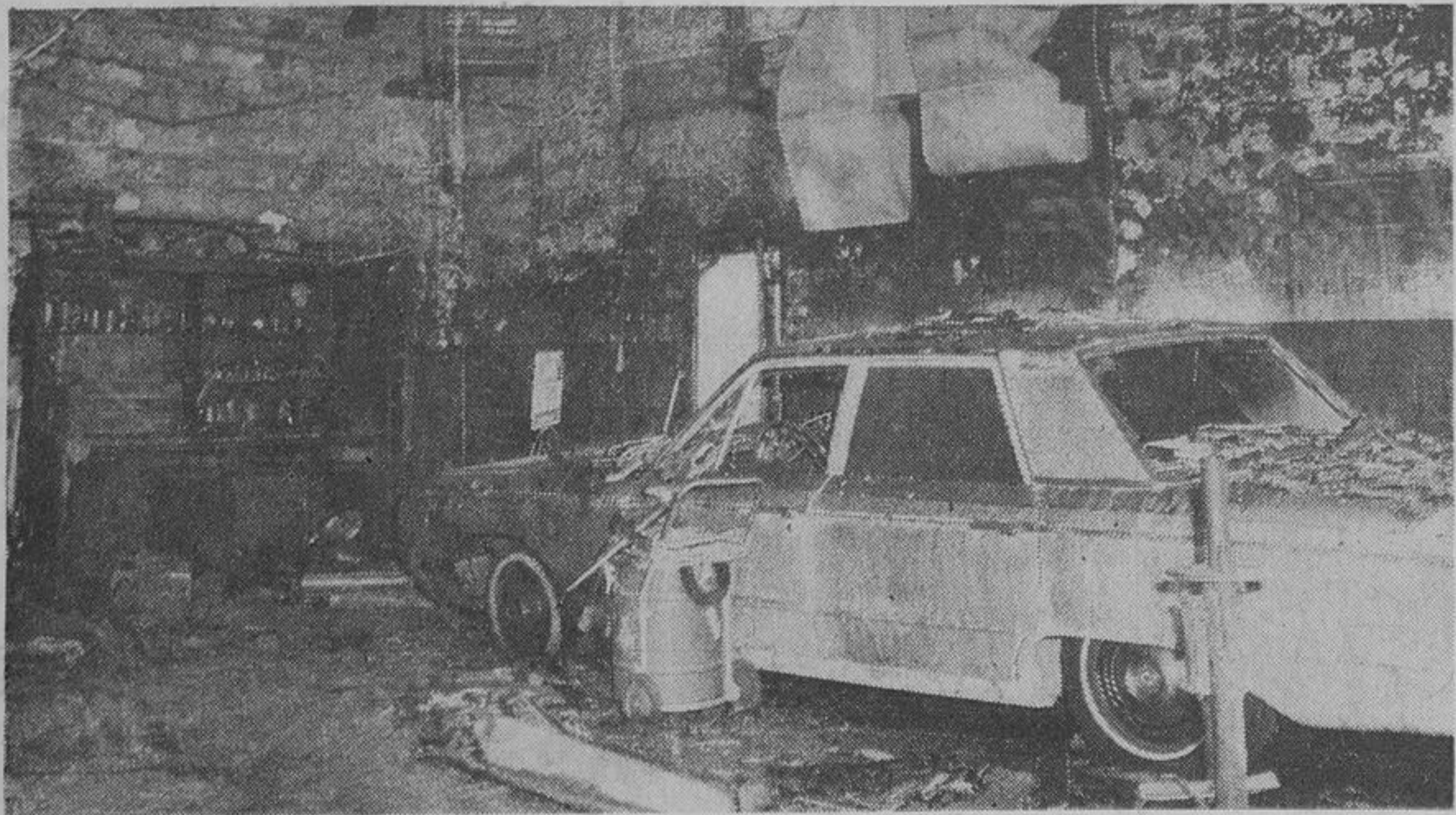
Gutted interior of the service station section of Sorenson Chrysler Highway 7, Concord, is seen after last Thursday evening's fire. The 1965 Dodge seen right, was completely destroyed. Damage is estimated at around $30,000.
