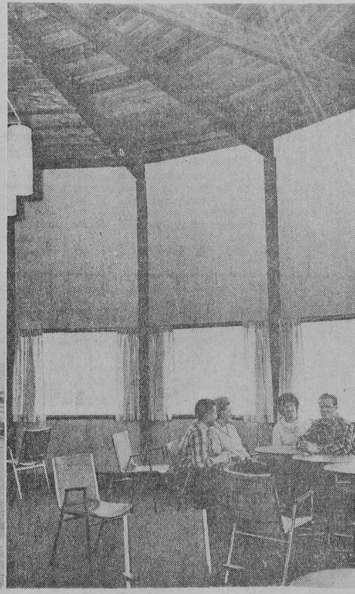
The tall circular tower of the executive lounge of the new quarters of the Port Credit Branch of the Royal Canadian Legion is not only unique in construction, but unique in location. Designed by King City architect Denis Bowman, the tower has as its foundation the old digester tank of the Port Credit sewage treatment plant.
