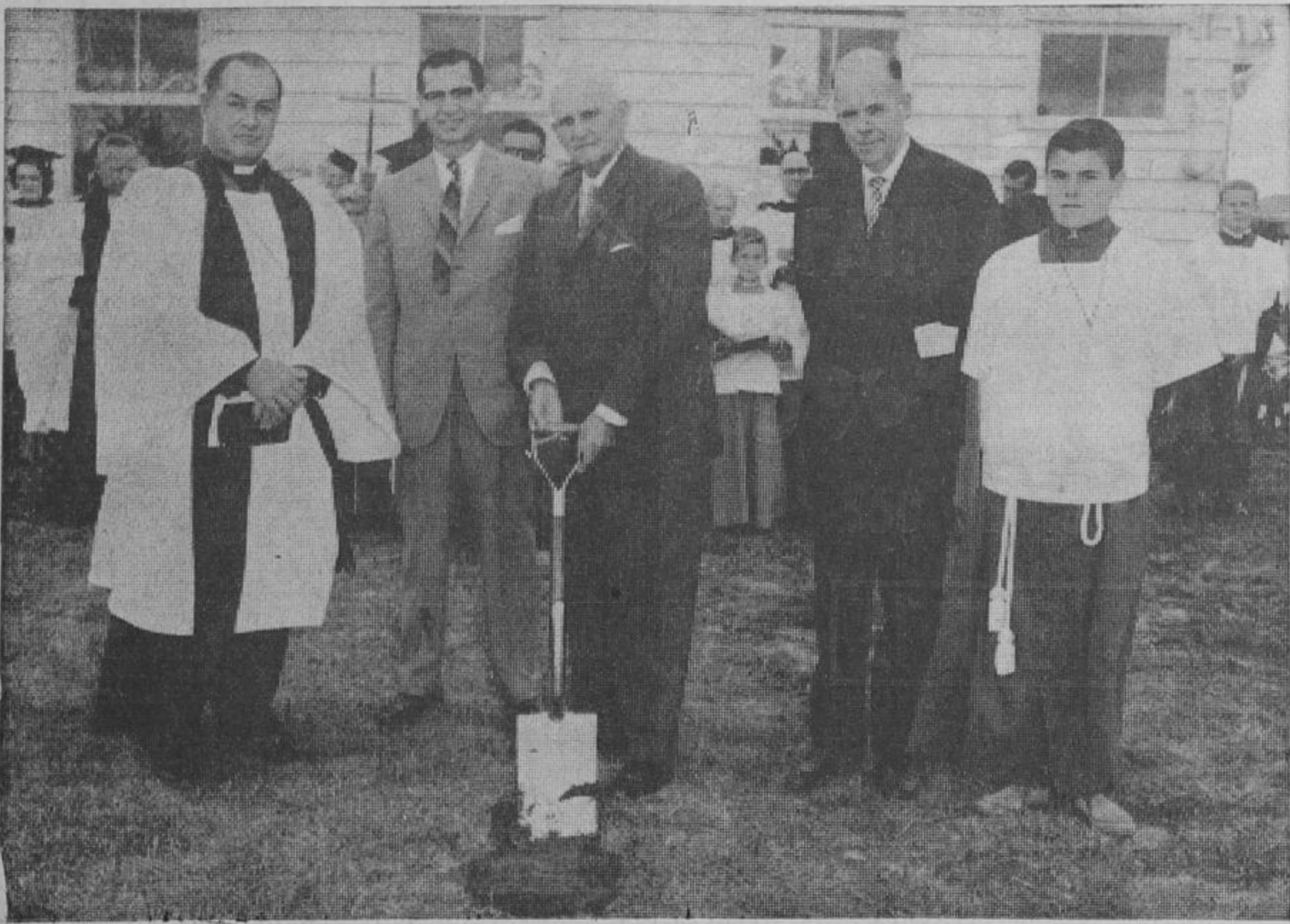
Pictured at the October 4 sod turning for the new Emmanuel Anglican Church on Mackay Drive, Richvale, are (left to right) Rev. K. Thatcher, Rector, G. Lunau, former warden, Henry Glover one of the founders of the original Emmanuel Church on Hanlan's Point, Leslie Walters, former warden, and Vernon Walters, servier.
