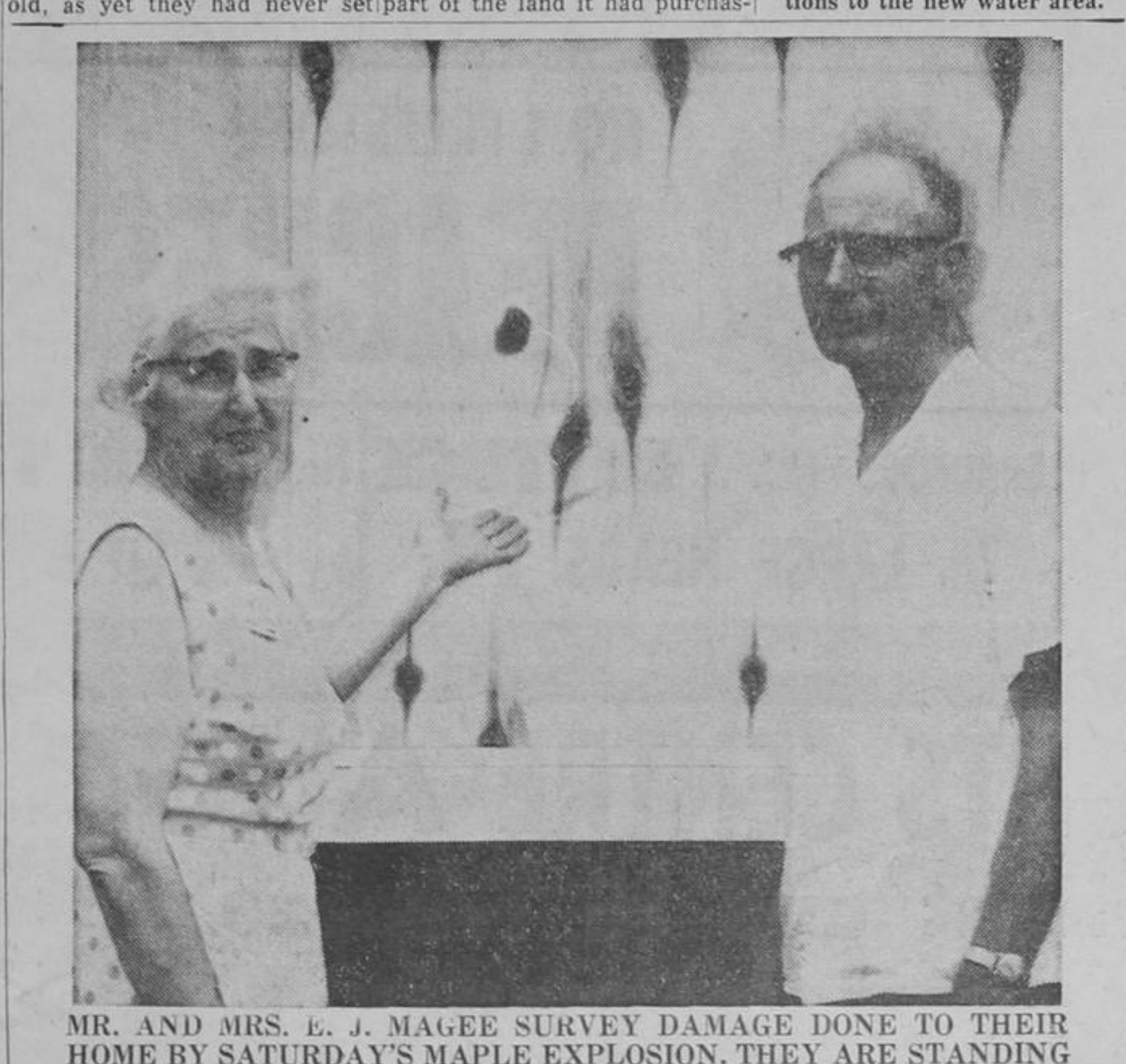
MR. AND MRS. E. J. MAGEE SURVEY DAMAGE DONE TO THEIR HOME BY SATURDAY'S MAPLE EXPLOSION. THEY ARE STANDING IN FRONT OF THE PLYWOOD OVER THEIR LIVING ROOM WINDOW.
