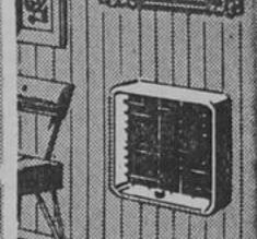
RADIANT WALL PANELS Radiant heating units, mounted into wall or ceiling,
