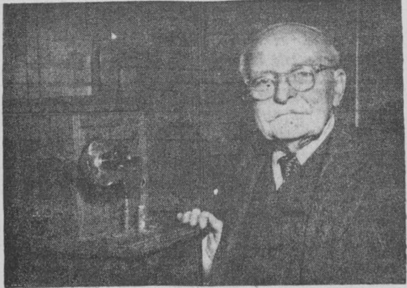
Alexander Bruce posed for this picture beside his company's first switchboard, which served ten lines. The company now serves 2,000 telephones.
