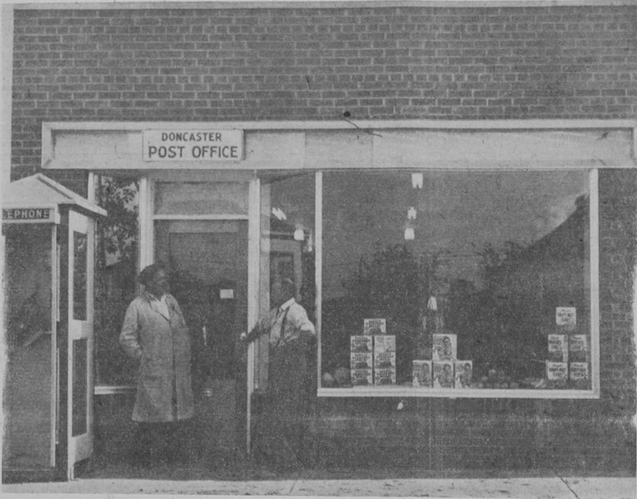
Here is the new and completely modern General Store conveniently situated at 59 Morgan Ave., Doncaster. Quality merchandise at low prices at all times will be a feature of this welcome addition to the commercial life of Doncaster. The owner and operator is Mr. Bert Richardson who places his talling business at the disposal of his friends and customers. A complete stock of groceries, meats, fruits and vegetables and drugs, will be handled by the store.
