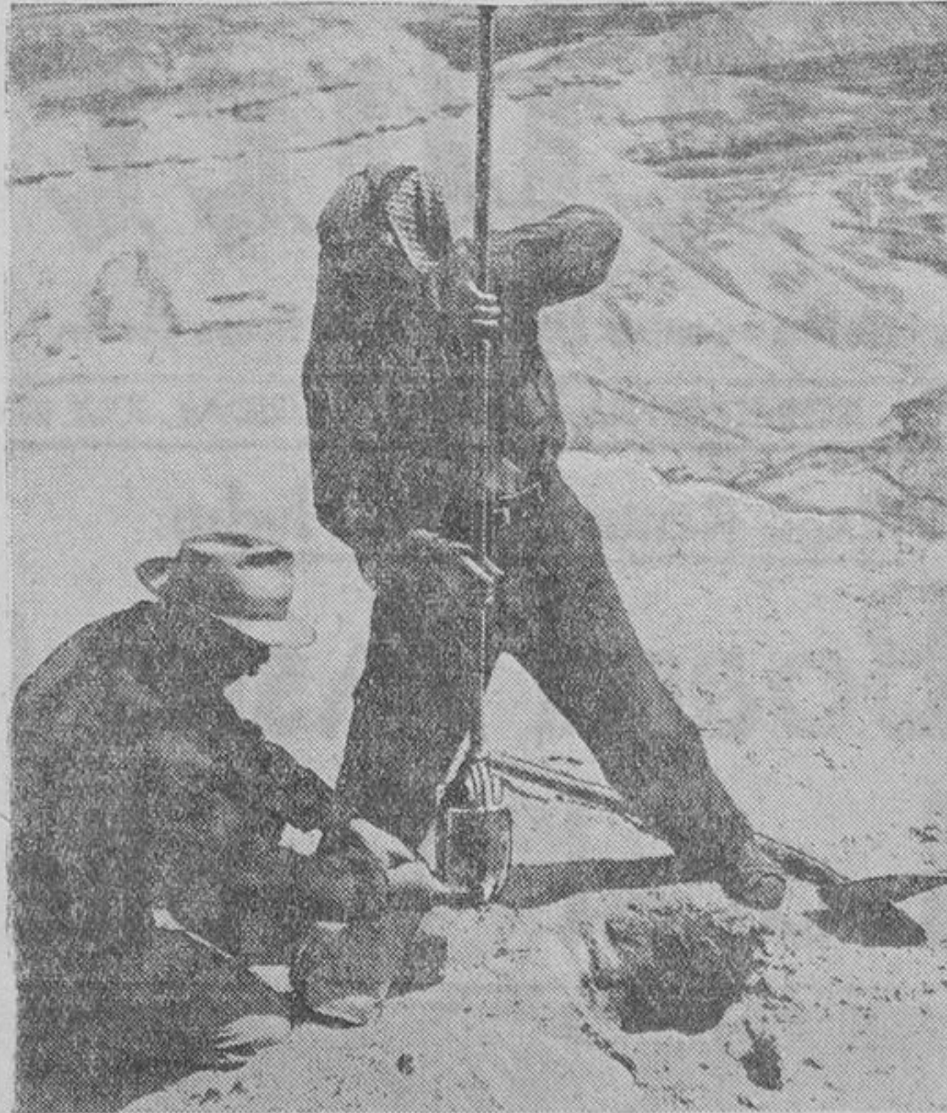
Examining a soil sample in the Jordan Valley, a water development expert (left) gathers data on irrigation possibilities. The United Nations Relief and Works Agency for Palestine Refugees recently agreed with the Kingdom of Jordan to provide $40,000,000 for construction of an irrigation and power dam in the region. The dry land, given water, might support up to 20,000 refugee families.
