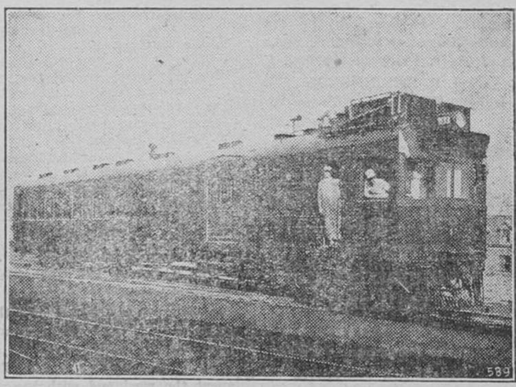
tors purring and humming in at an average speed of 30 miles soothing but powerful harmony, an hour, but attain a maximum No. 47, the Canadian Pacific Railway's new gas-electric combined passenger and baggage car, embodying the latest developments in electro-motive traction, travels smoking compartment for 15 peobetween Hamilton and Goderich ple and a 17-foot compartment and its sister car No. 46, between for baggage and express.
