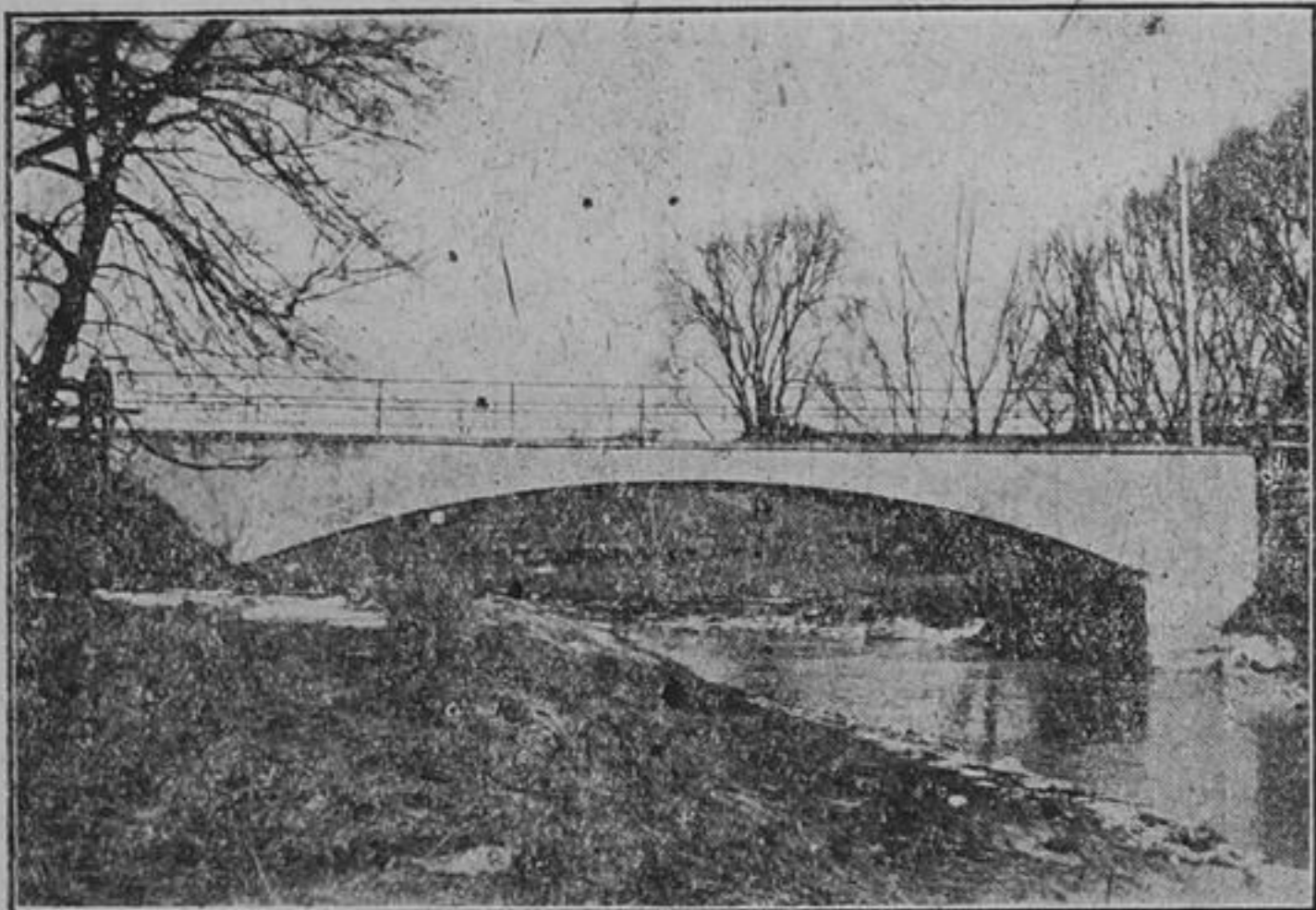
First Concrete Bridge in York Erected 1908, Enlarged 1926.
