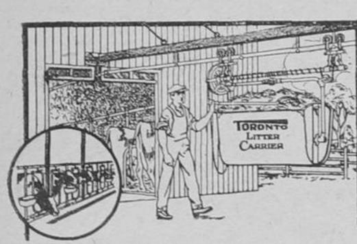
With one of my Toronto Litter Carriers, one man can clean your stable as fast as three in the old way. Do it, too, without the unpleasantness and muss of the wheelbarrow method. Dump the manure into a pile
