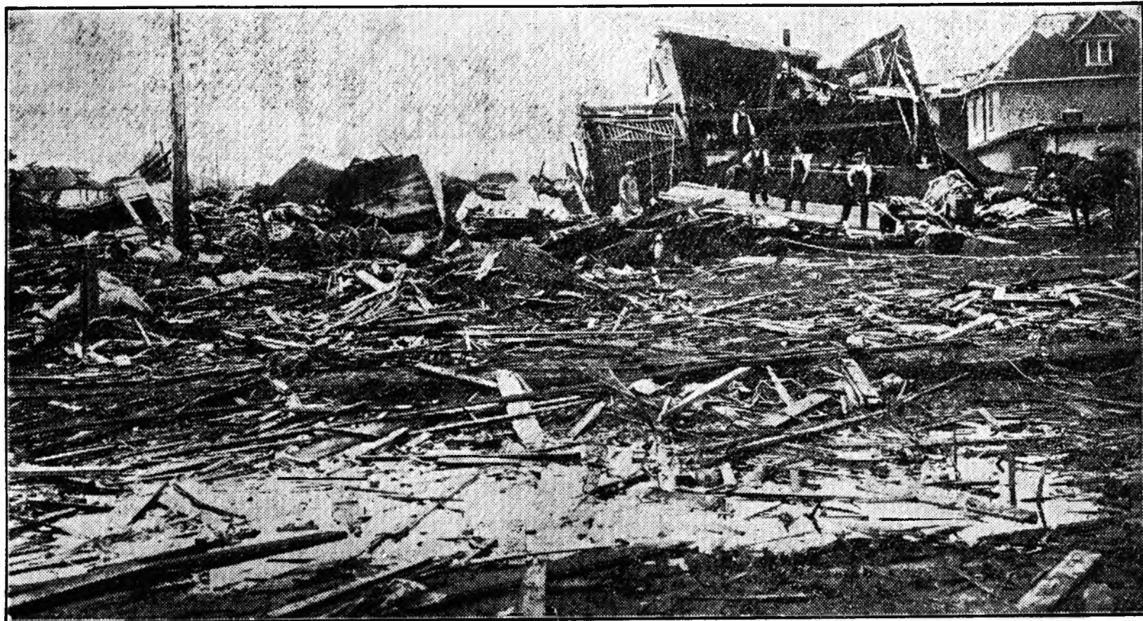
Portion of the ruins of Smith Street south. This and Lorne Street were wiped clean from end to end—two miles of ruin.
