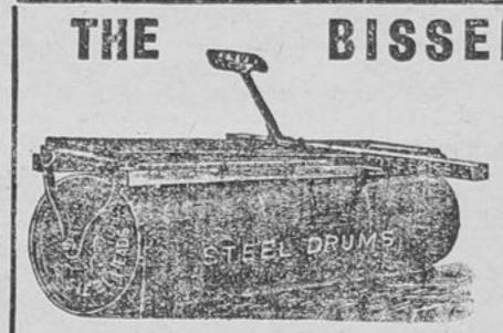
With Three Drums and Strong, Rigid Frame. ome improvements are: Heavy Steel Axle, hick, Heavy Steel Plate, Drums Rivetted up stand any strain, Roller Bearings. Runs like a bird. Full particulass free by mail, or ask your dealer. None genuine without the name "BISSELL." For Sale by Agents.
